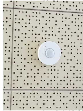
Ceiling Mounted Occupancy Sensor
