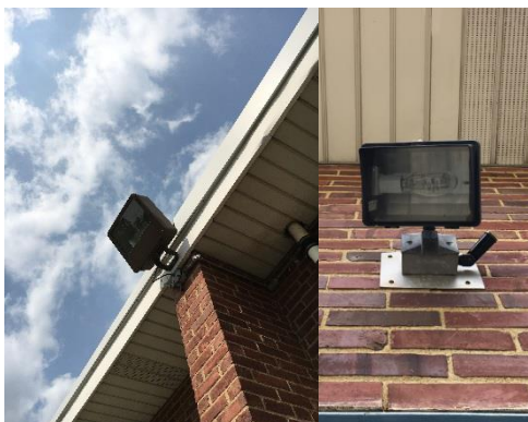
HID Wall Mounted Flood Fixtures
