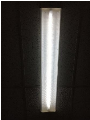
Surface Mounted Wrap Fixtures
