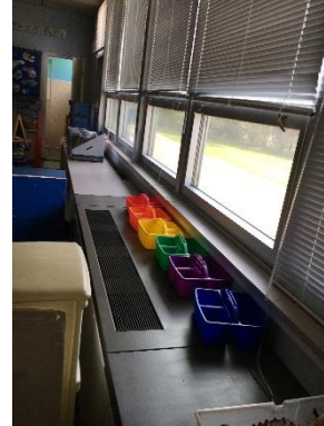
New Unit Ventilator
