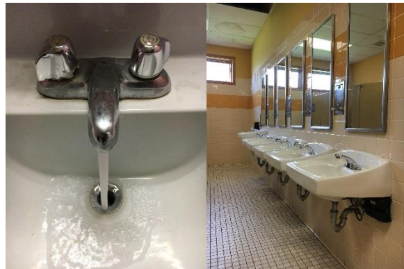
High Flow Aerator and Low Flow Sinks
