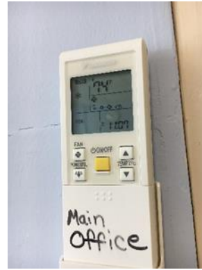
Split AC System - Remote
