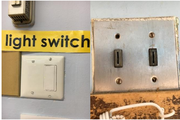
Wall Switch and Key Switch
