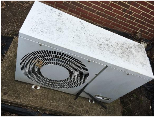
Split AC Systems – Outdoor Condensing Unit
