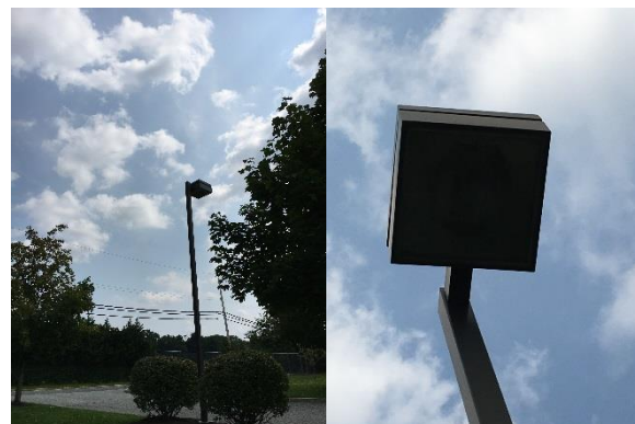
HID Pole Mounted Shoe Box Fixture
