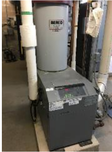
Image 5 Domestic Hot Water Heating System
