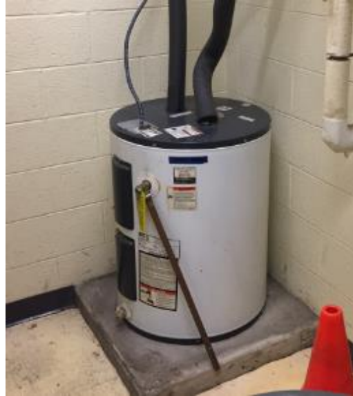
Image 15. Picture of the Electric DHW Water Heater
