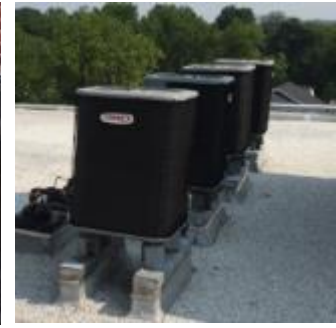
Image 11. Picture of Lennox Condensing Units serving Unit Ventilators
