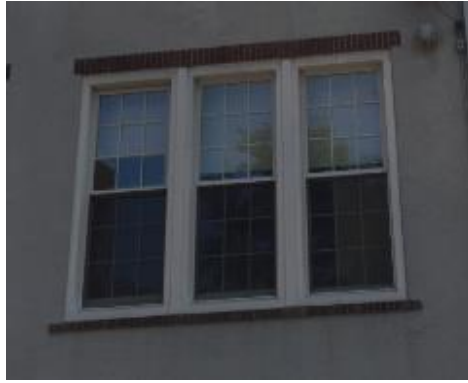
Image 4. Picture of a Window in an Older Section of the Building
