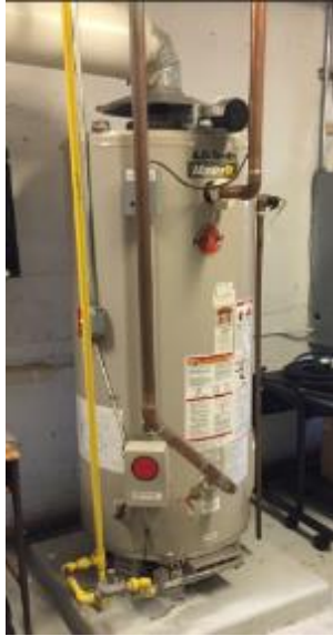
Image 14. Picture of the Gas DHW Water Heater
