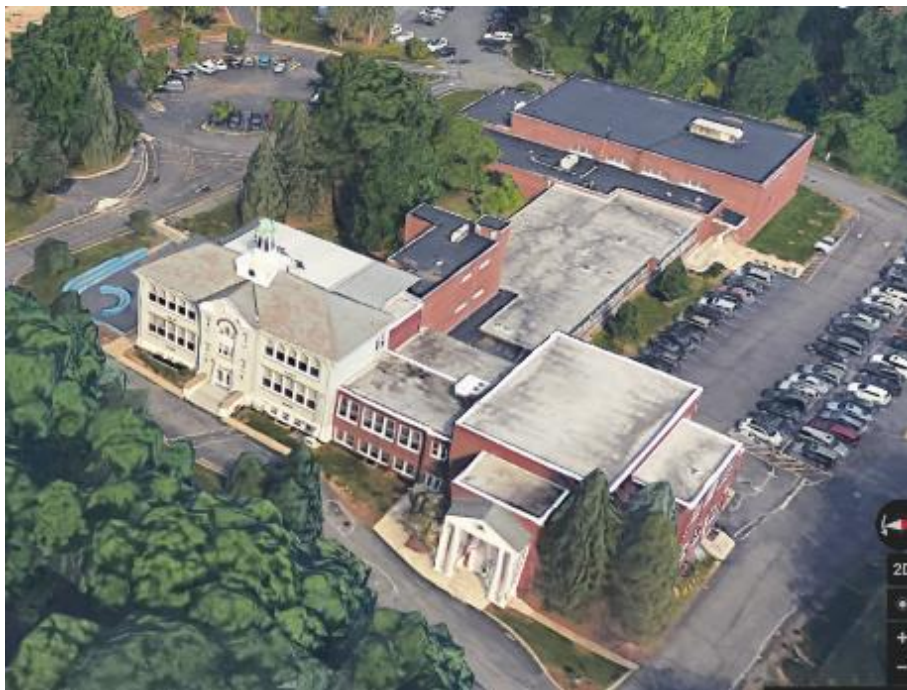
Image 1: Aerial screenshot of the building
