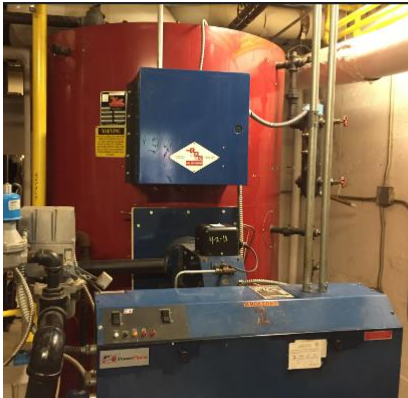
Image 12. Picture of Steam Boiler
