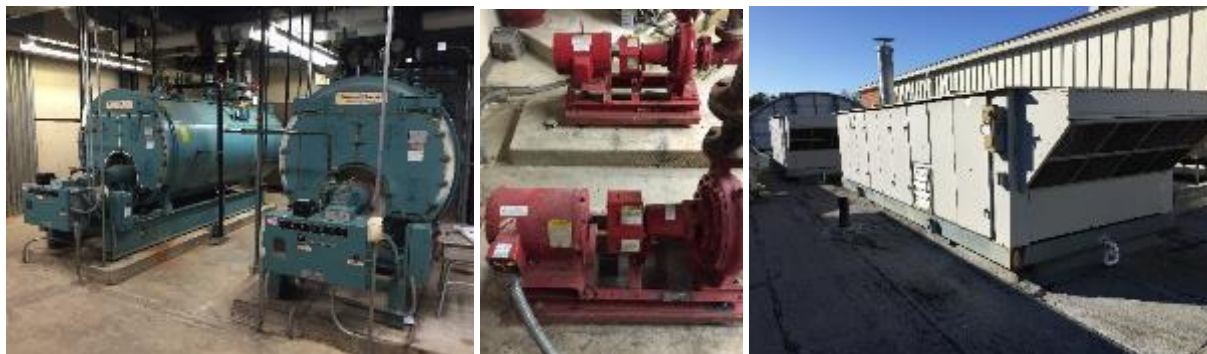
Image 3: Heating and Ventilation Systems
