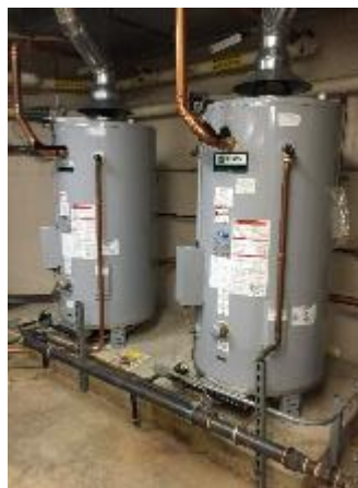
Image 5: Domestic Water Heating
