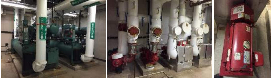
Image 4: Chiller and Chilled Water Distribution
