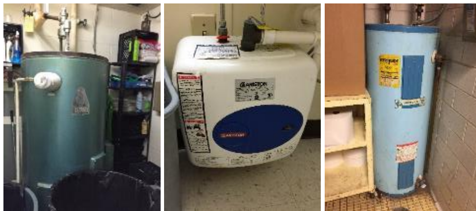
Image 4: Domestic Water Heating Systems
