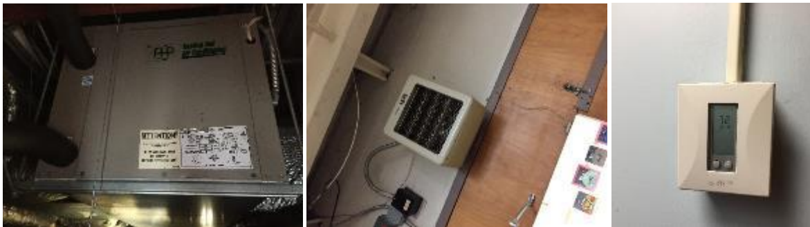
Image 3: Air Conditioning and Heating Systems
