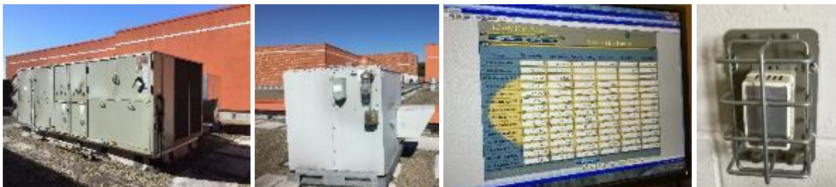
Image 3 Heating and Air Conditioning System
