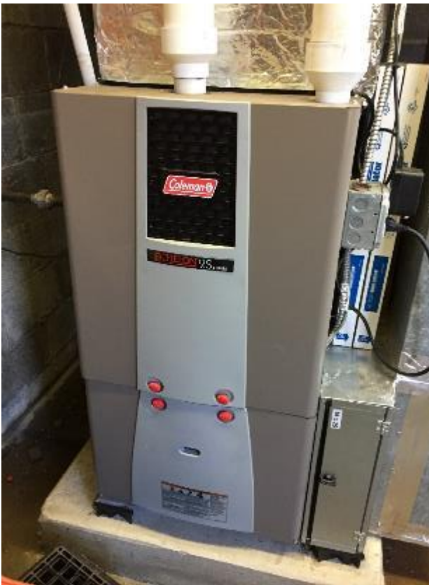
Image 7 – AHU w/Gas Furnace (Annex)
