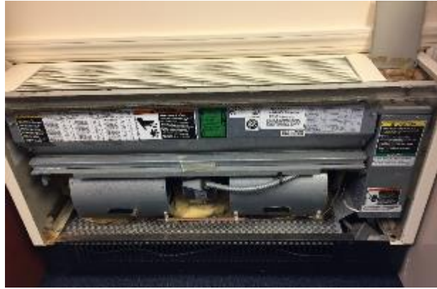
Image 6 – Through-Wall AC (Admin)
