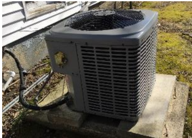
Image 8 – Programmable Thermostat & Split System Condenser (Annex)
