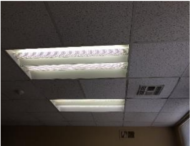
Image 3 – General Lighting (Annex)
