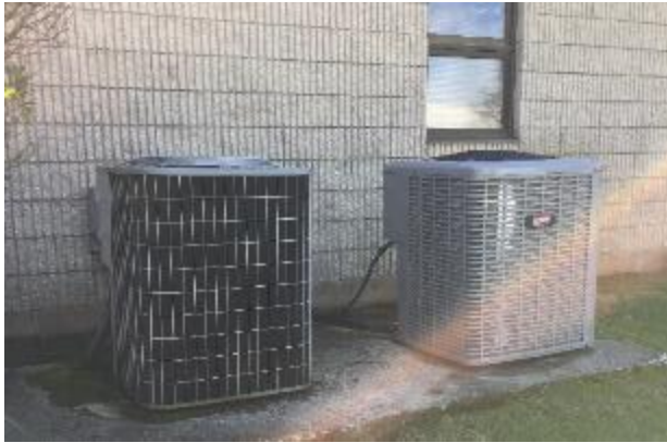
Image 5 – Heat Pumps (Admin)
