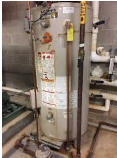
Image 6: Domestic Water Heating System
