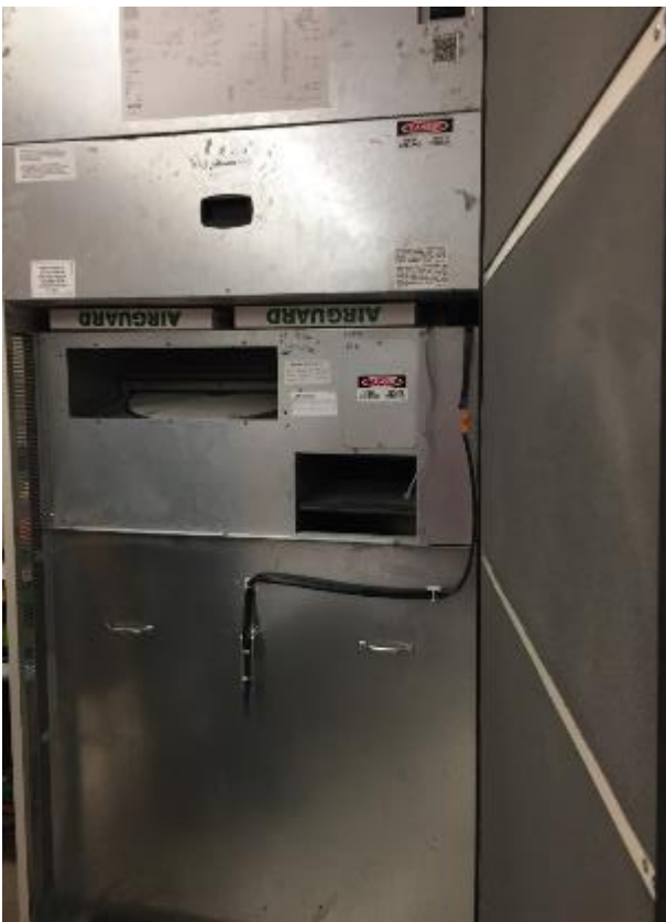
Image 6 In-classroom package unit w/HW coil
