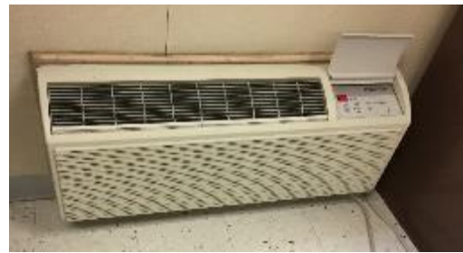
Figure 4: DX Cooling Systems
