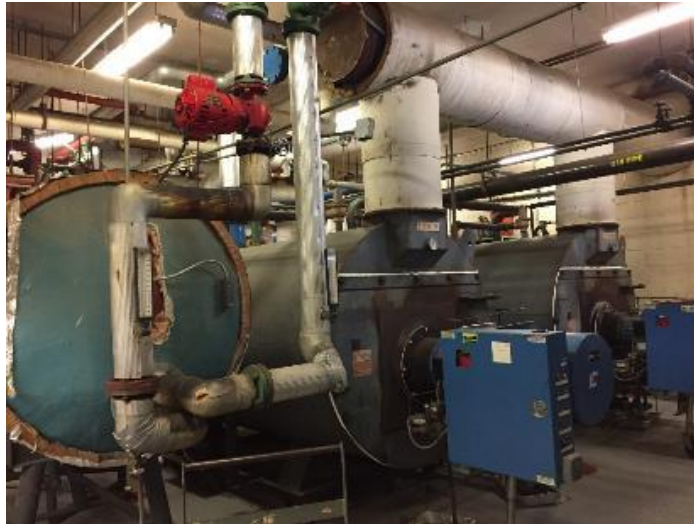
Figure 3: Hot Water Heating Systems
