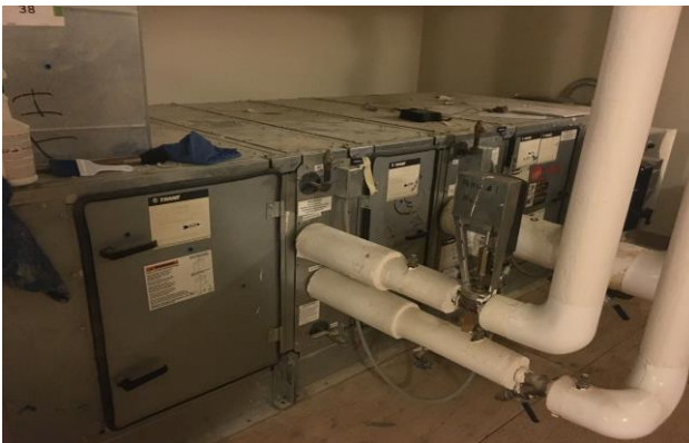
Image 5: Air Handler (AHU-1)
