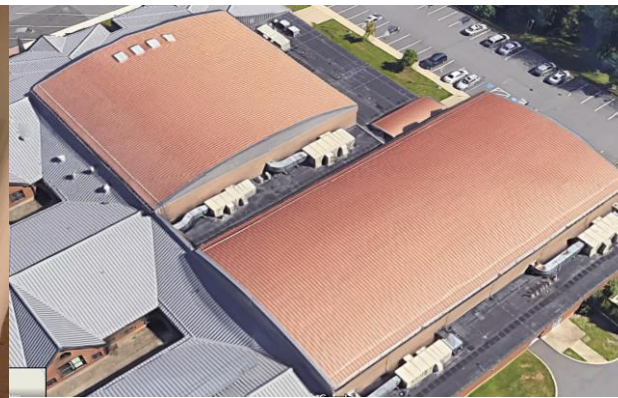
Image 6: Roof-top Units over Gym and Cafeteria
