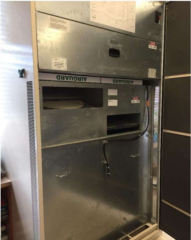
Image 8 In-classroom package unit w/HW coil
