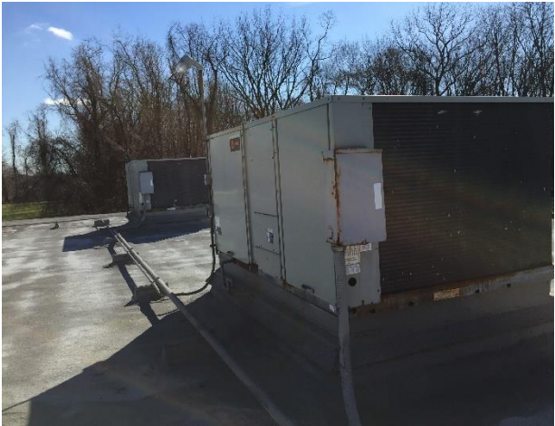
Image 6 Packaged DX units serving Cafeteria
