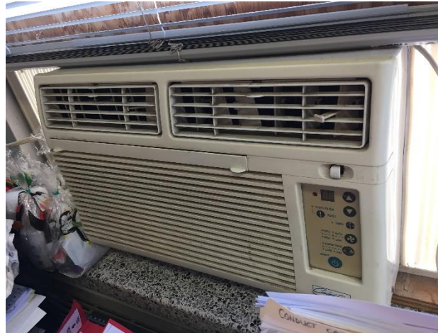
Image 7 Typical window AC unit
