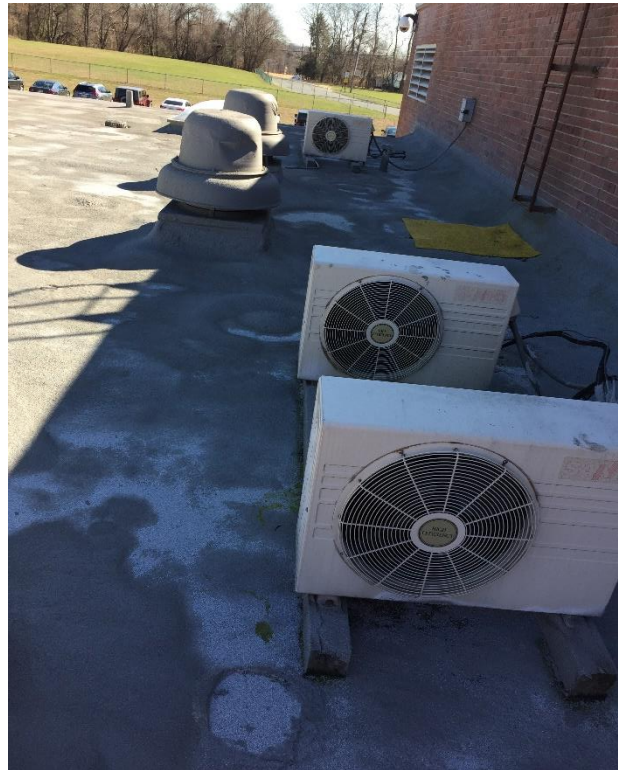
Image 9 Split System outdoor units (condensers)
