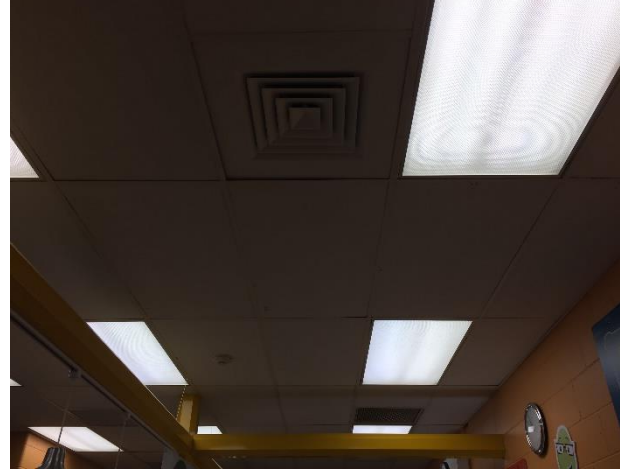
Image 3 Typical classroom lighting
