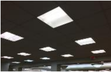
Image 8. Troffer Fixtures with CFL Long Lamps
