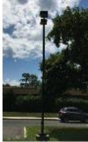
Image 11. Pole Mounted Fixtures
