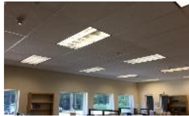
Image 6. Linear Fluorescent Troffer Fixtures
