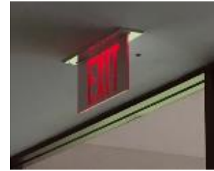
Image 10. LED Exit Sign
