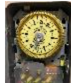
Image 14. Exterior Lighting Control Timer
