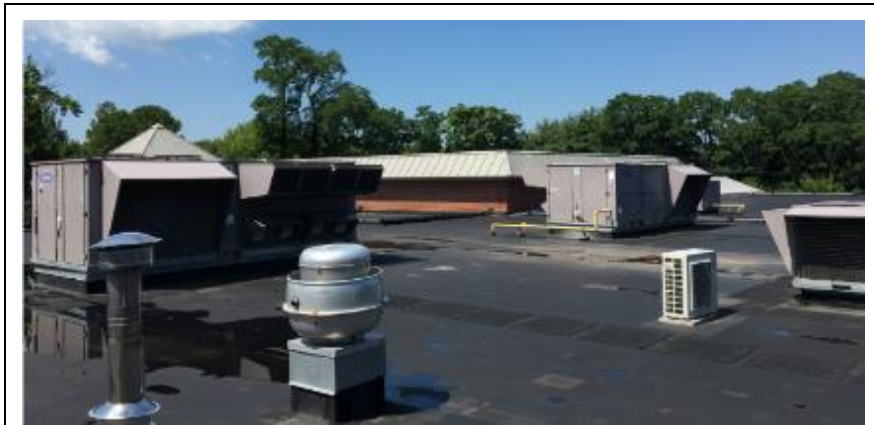
Image 15. Picture of Rooftop Package Units and Heat Pump Condenser Unit
