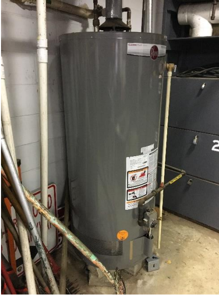
Image 17 – 75 gallon gas-fired water heater
