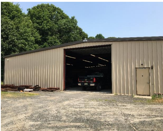
Image 3 – Municipal Garage envelope
