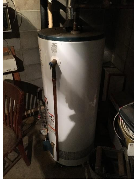
Image 18 - 40 gallon gas-fired water heater
