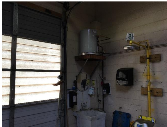
Image 19 – 2kW electric water heater
