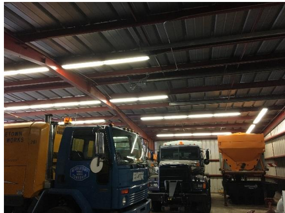
Image 6 – Garage 1 linear fluorescent fixtures
