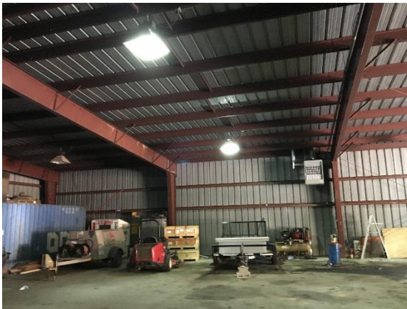
Image 5 – Garage 2 metal halide fixtures
