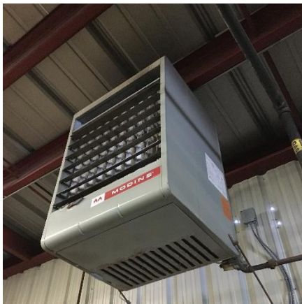
Image 13 – Municipal Garage gas-fired unit heater
