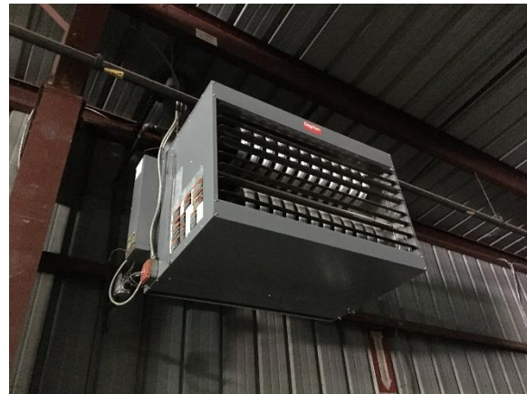
Image 14 – Municipal Garage gas-fired unit heater
