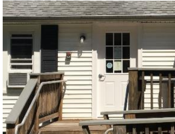
Image 4 – Exterior metal door
