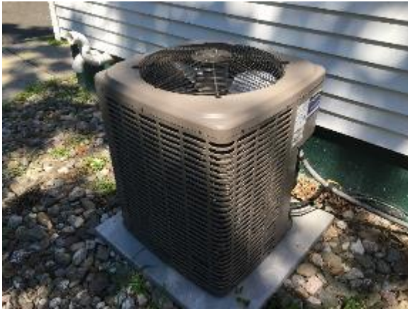
Image 9 – AC condensing unit
