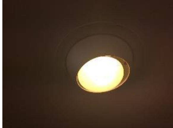
Image 6 – Recessed can fixture
