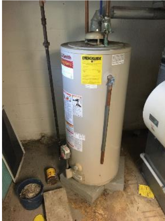
Image 13 – Domestic Water Heater
