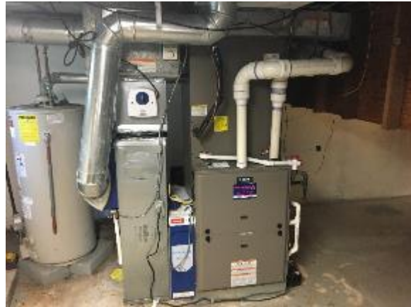
Image 10 – Air handling unit w/AC evap coil & furnace
