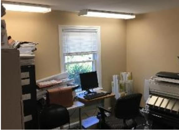
Image 5 – Typical surface mounted T8 fixtures
