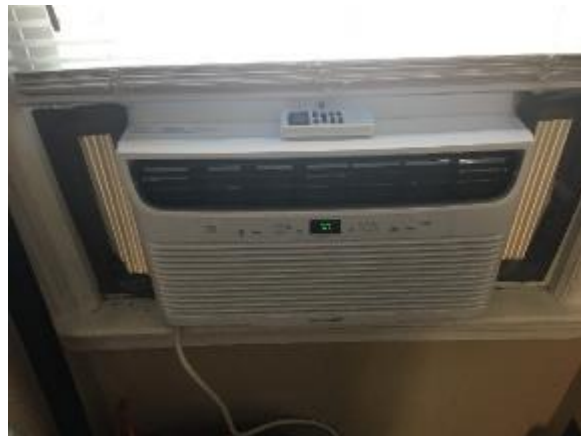
Image 12 – Window AC (office)
