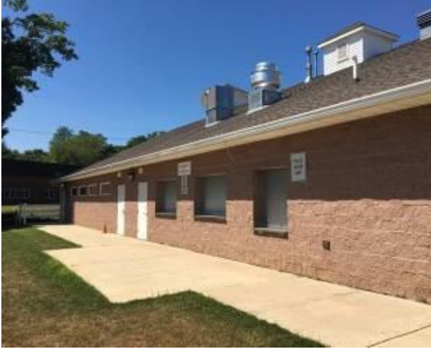
Field-side of building
