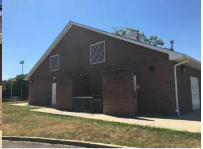
Side of building
