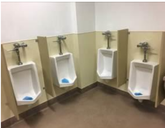
Men's Restroom - Urinals
