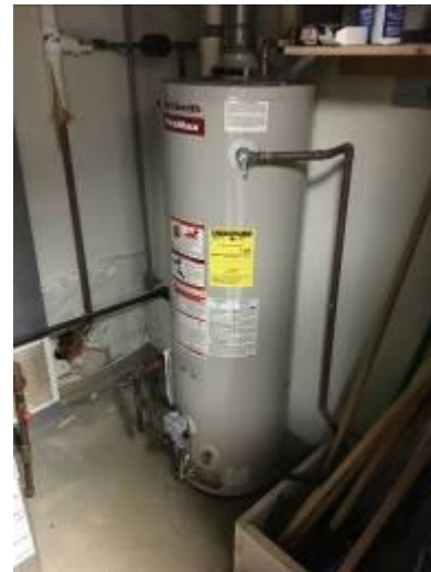
McMahon Park – Water Heater
