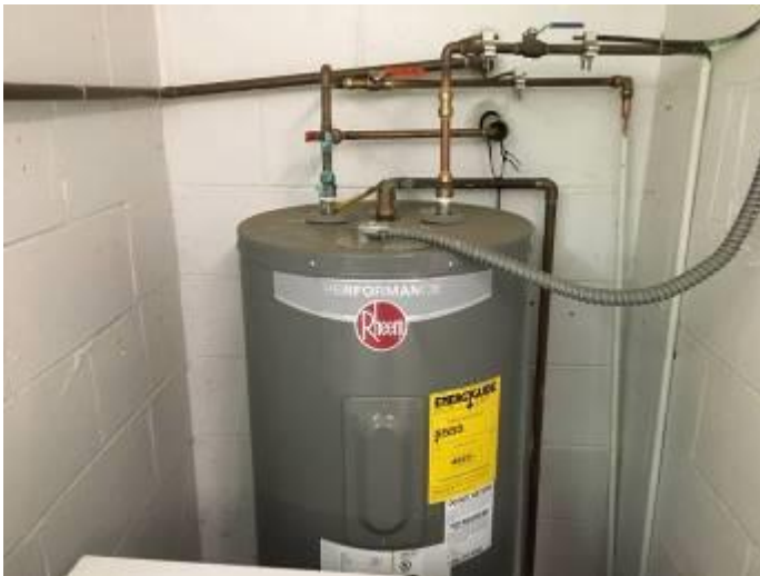
Nick Trezza Bldg.- Water Heater
