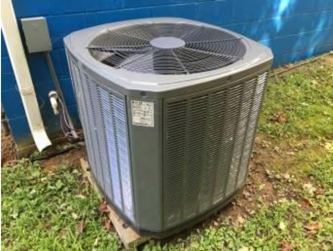
Nick Trezza Field Cottage - Split System AC
