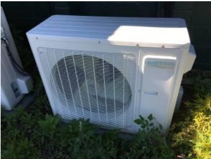
Bodman Park MYAA Building – Mini-Split HP
