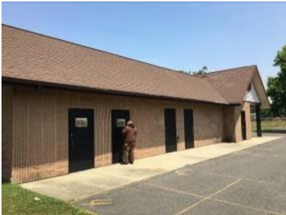
McMahon Park Concessions Building
