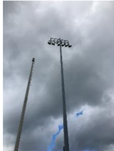
Nick Trezza Field MH Fixtures
