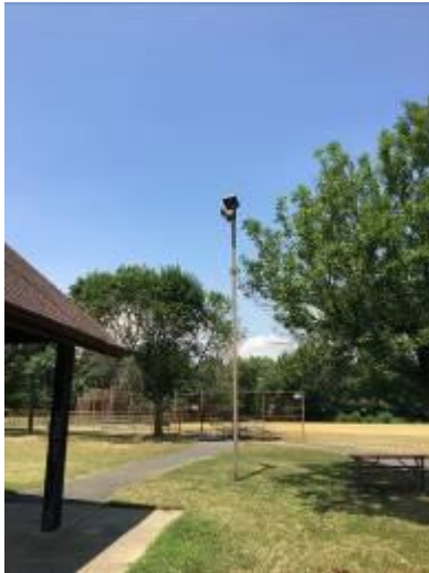
McMahon Park MH Fixtures
