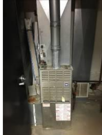
McMahon Park Bldg– NG Gas Furnace
