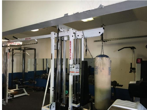
Image 6 – Gym recessed T8 fixtures
