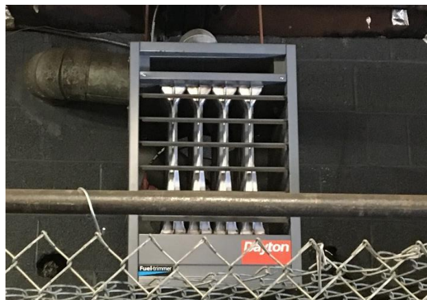
Image 12 – Storage unit heater
