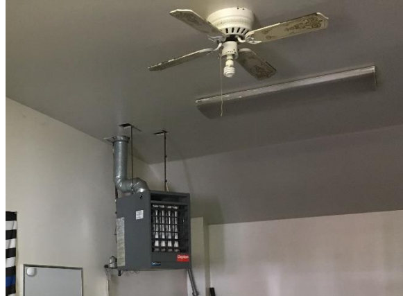
Image 14 – Gym ceiling fan
