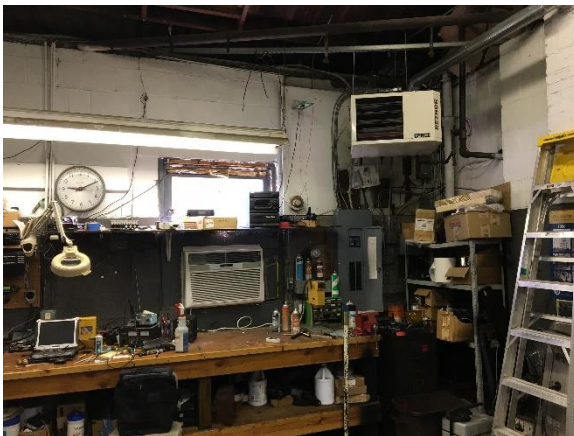
Image 7 – Suspended T12 fixture in Radio Repair
