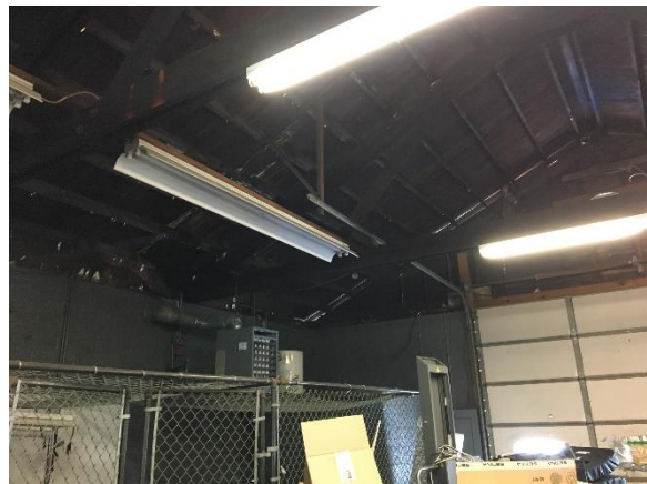
Image 8 – Surface mounted T12 fixtures in bay
