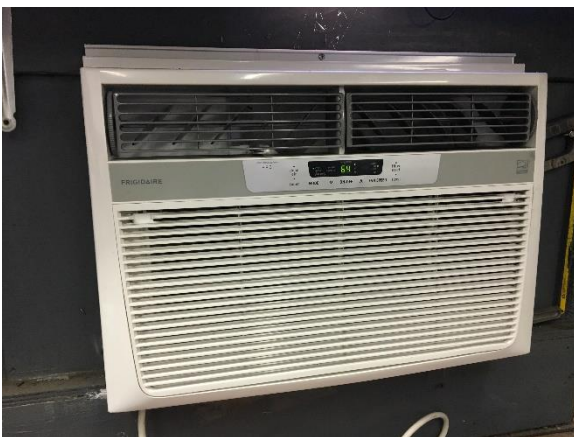
Image 11 – Radio Repair AC unit
