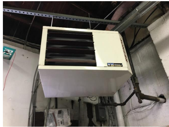
Image 10 – Radio Repair unit heater
