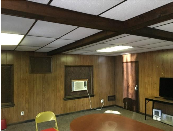
Image 5 – Classroom recessed T8 fixtures
