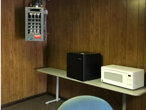
Image 13 – Classroom mini-fridge & microwave
