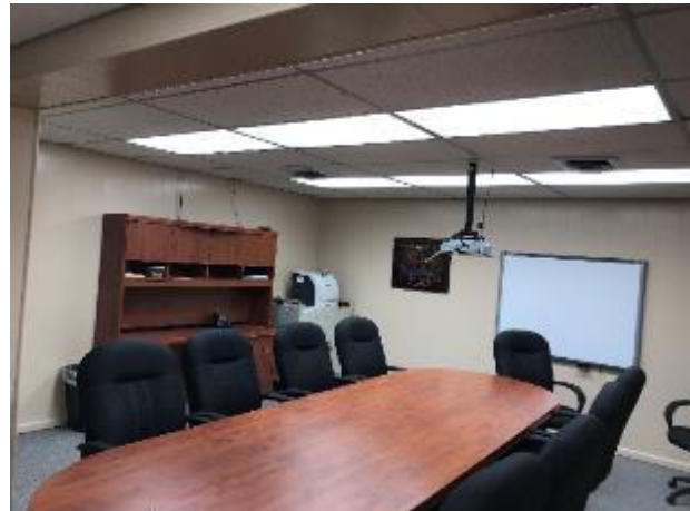
Image 8 Conference Room Lighting
