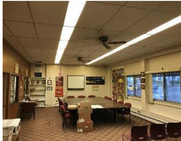
Image 6 Conference Room Lighting
