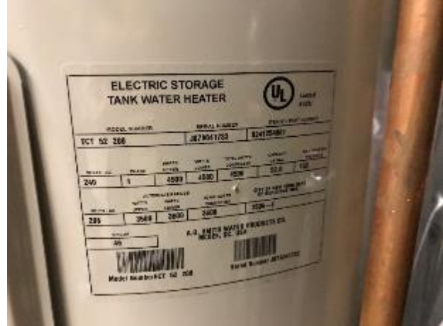
Image 26 Hot Water Heater Nameplate
