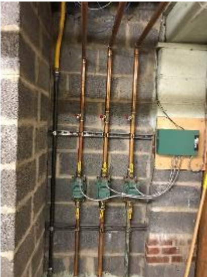
Image 23 Hot Water Pipes Without Insulation
