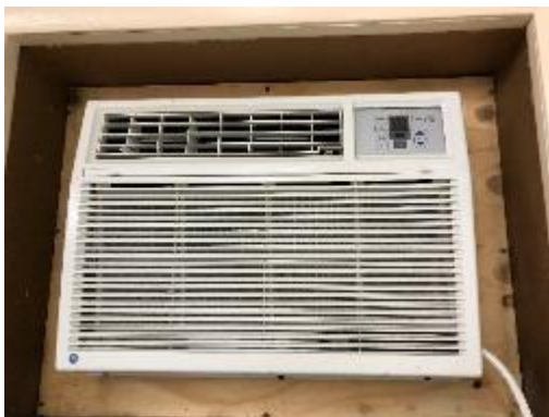
Image 19 Window AC in Facility Office
