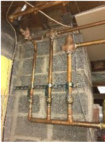
Image 27 DHW Pipes Without Insulation
