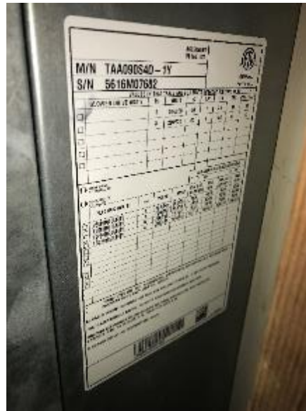
Image 16 Split system AC Nameplate
