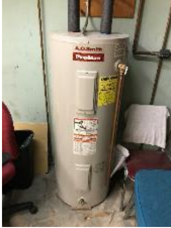
Image 25 Hot Water Heater
