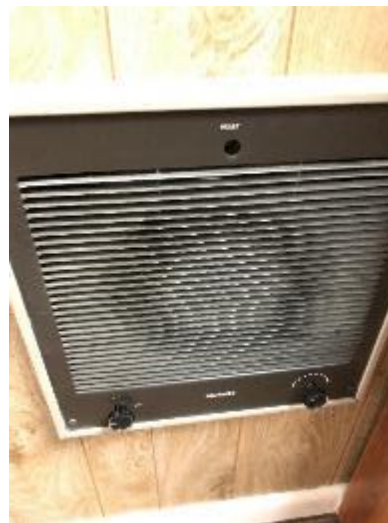
Image 20 Wall Mounted Heater
