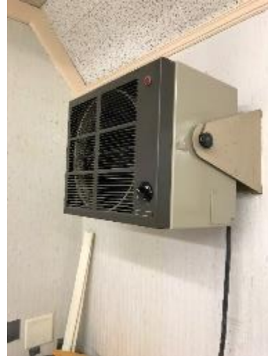
Image 18 Electric Heater in Facility Office
