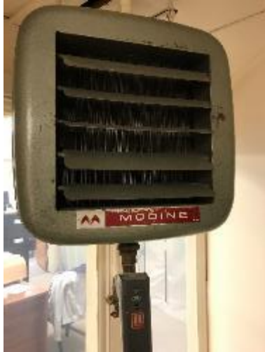
Image 17 Unit Heater in Basement
