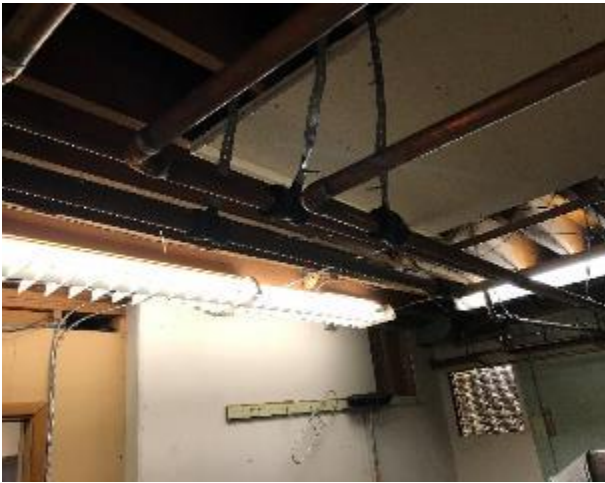
Image 5 Mech Room Lighting
