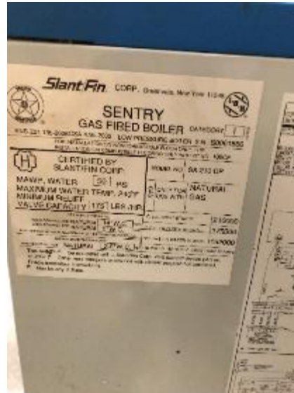
Image 24 Boiler Nameplate
