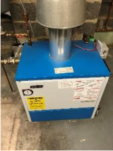
Image 21 Hot Water Boiler
