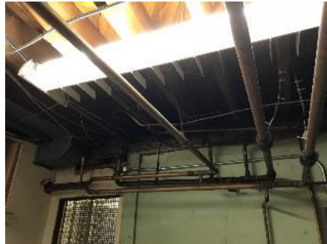
Image 28 Pipes Without Insulation
