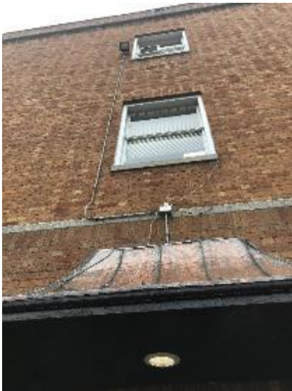
Image 11 Exterior HPS Fixture
