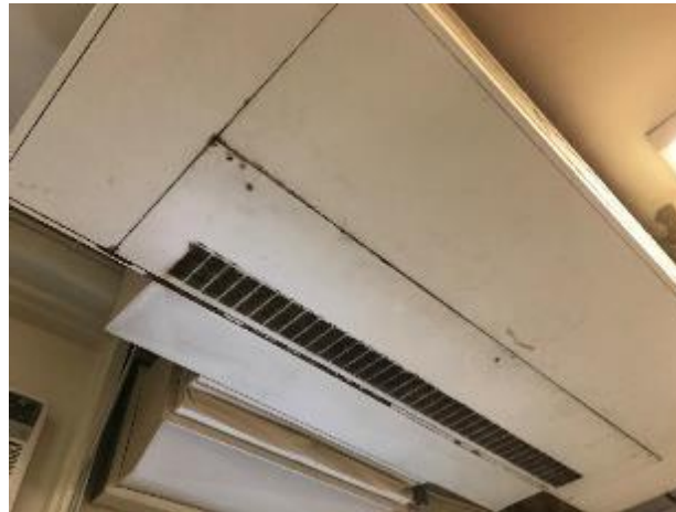
Image 16 Ceiling Mounted Unit Ventilator
