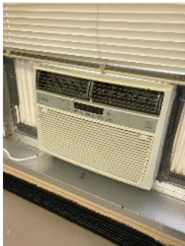
Image 23 Window AC in Classroom
