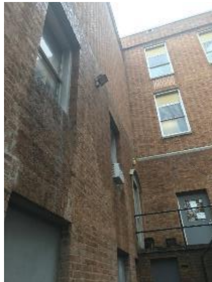
Image 12 Exterior HPS Fixture Type 2
