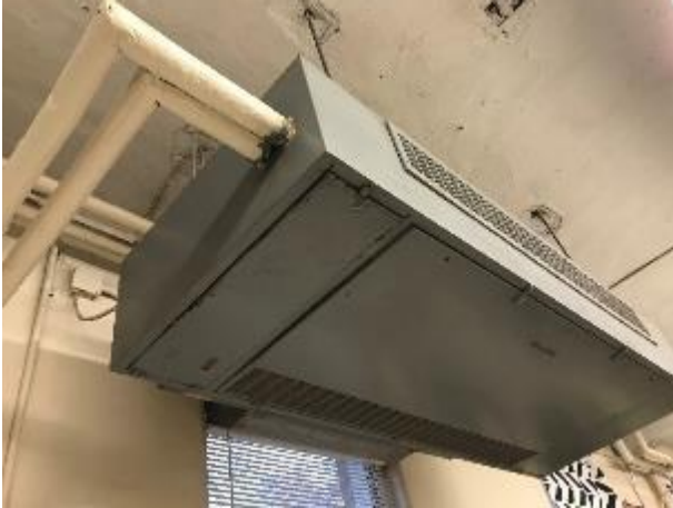
Image 13 Ceiling Hung Unit Ventilator
