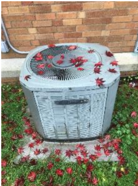
Image 19 Trane Outdoor Unit
