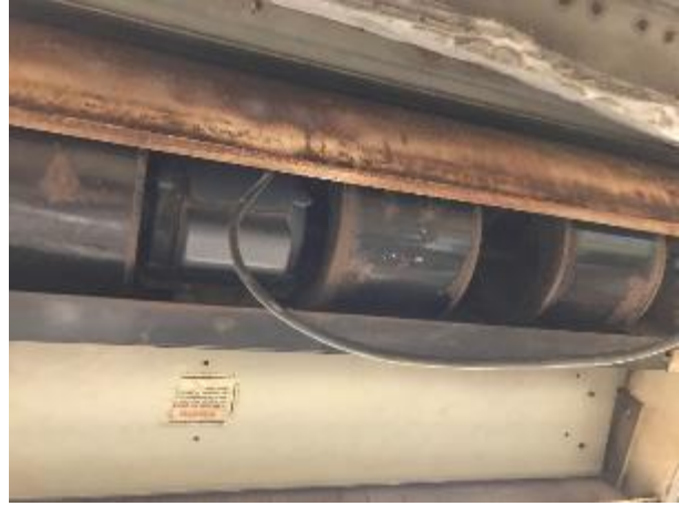
Image 14 Unit Ventilator Motor
