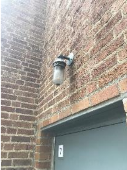
Image 9 Exterior Incandescent Fixture
