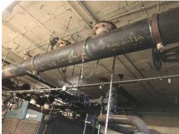
Image 26 Exposed boiler pipes
