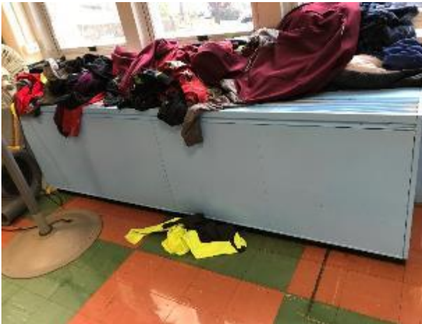
Image 15 Classroom Unit Ventilator
