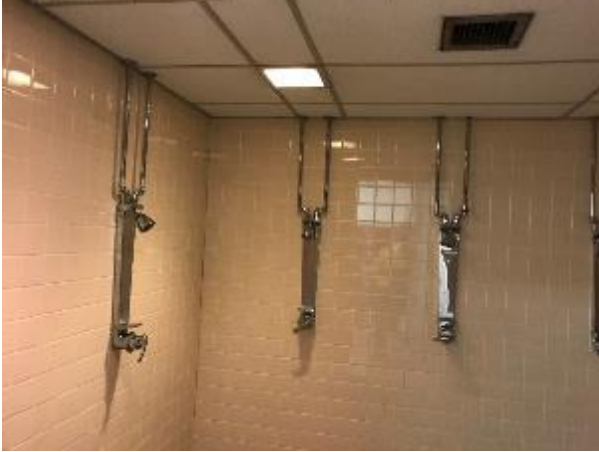
Image 41 Showerheads in Locker Room
