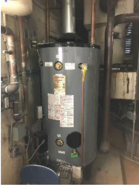
Image 29 Hot Water Heater
