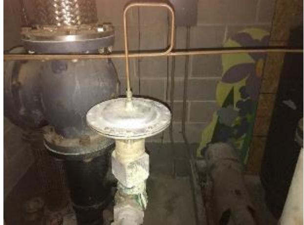
Image 18 HHW Secondary Pumps
