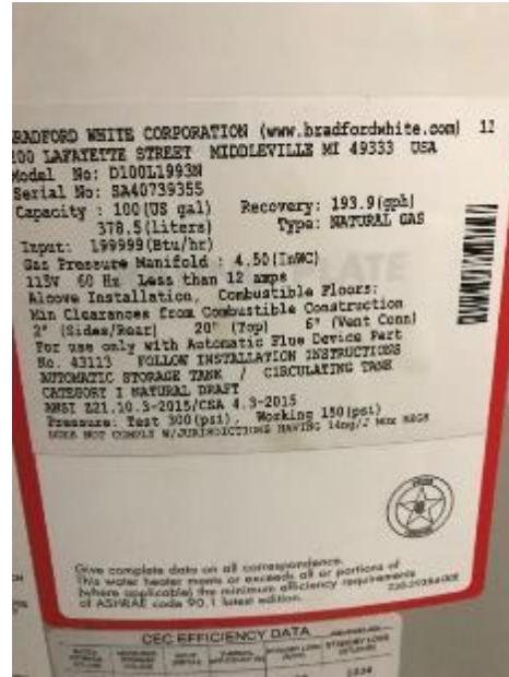
Image 26 Hot Water Heater Nameplate
