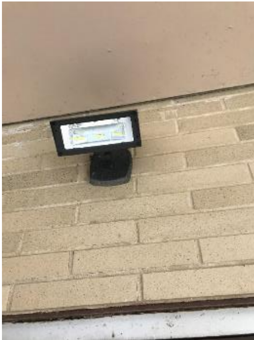
Image 11 Exterior LED Fixture
