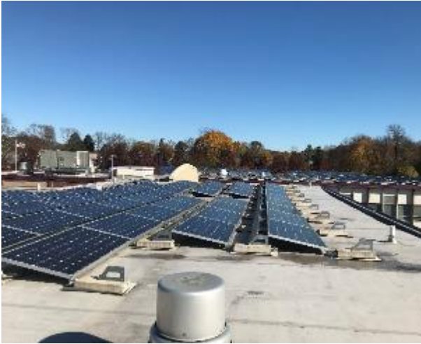
Image 37 Solar Panels on Roof
