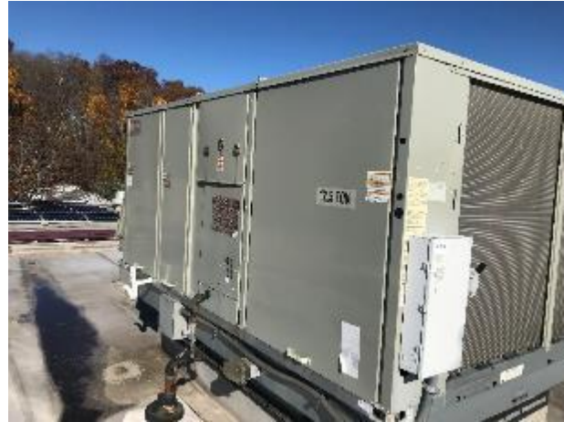
Image 14 Trane RTU Unit
