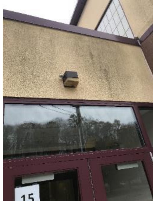
Image 10 Exterior CFL Fixture
