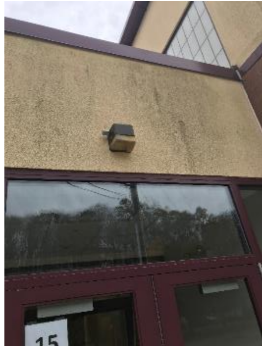
Image 12 Exterior Metal Halide Fixture
