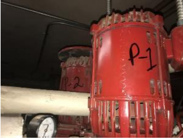
Image 17 HHW Primary Pumps
