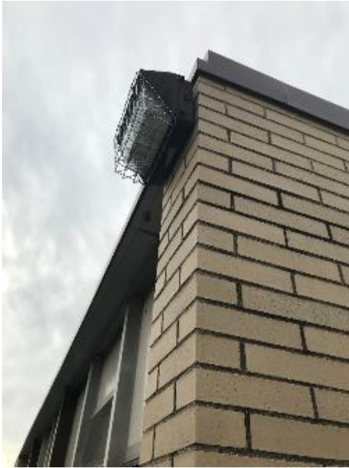
Image 9 Exterior HPS Fixture
