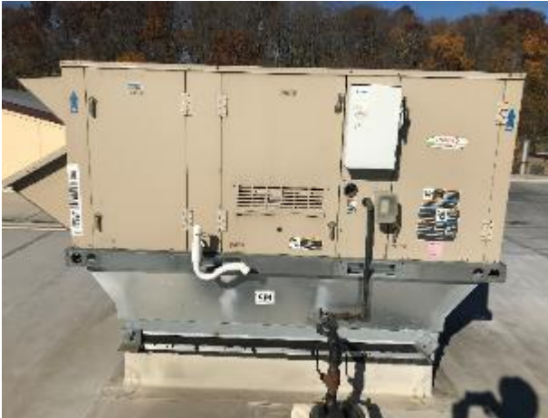
Image 13 RTU Lennox Unit
