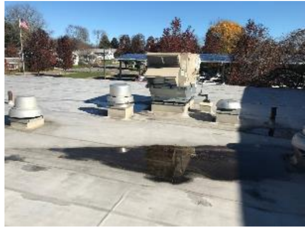
Image 16 RTUs on Roof
