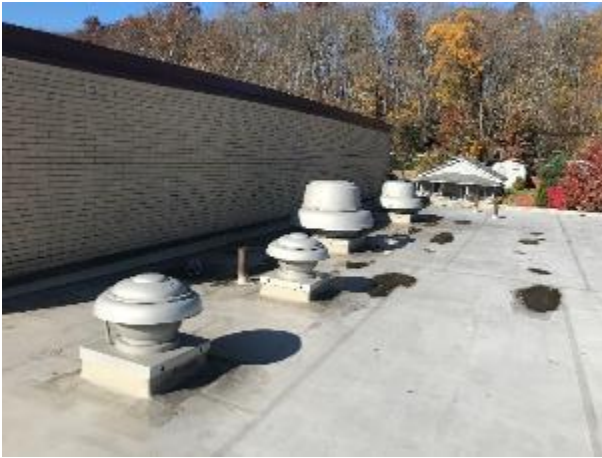
Image 15 Exhaust Fans on Roof
