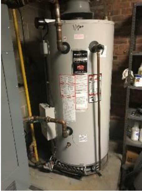
Image 25 Hot Water Heater
