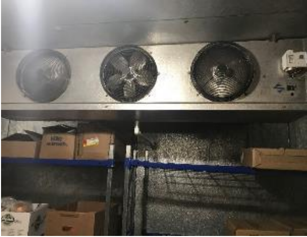
Image 33 Walk in Cooler Evaporator Fans
