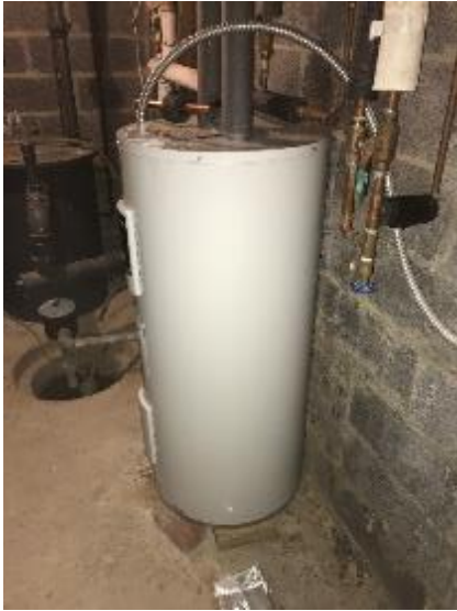
Image 25 DHW Storage Heater
