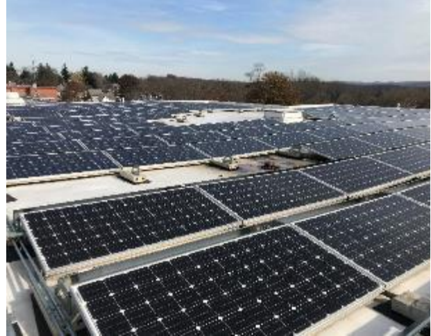
Image 46 Closer look at Solar Array
