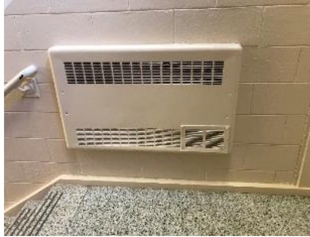
Image 18 Unit Ventilator
