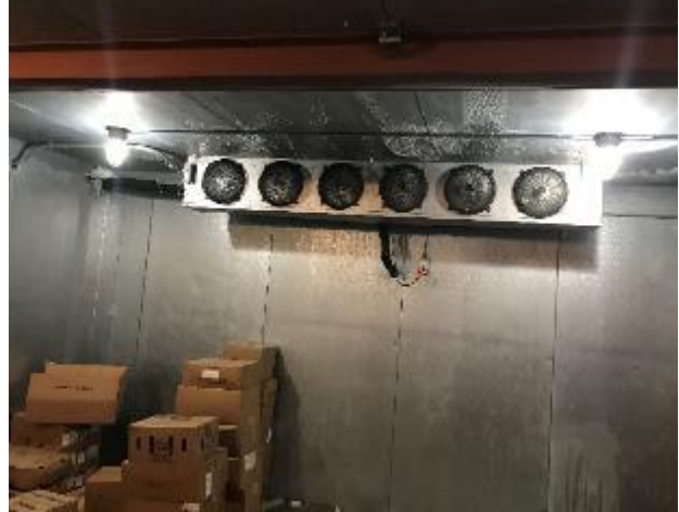
Image 34 Walk in Freezer Evaporator Fans
