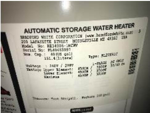
Image 27 DHW Heater Nameplate
