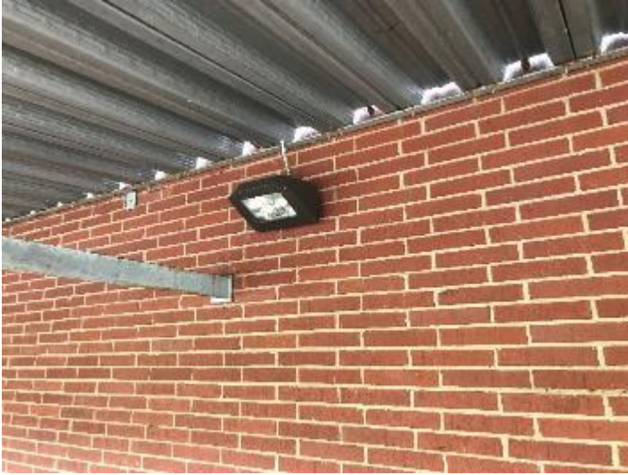
Image 13 Exterior LED Wall Pack Fixture
