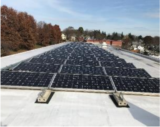
Image 45 Solar Panels on Roof
