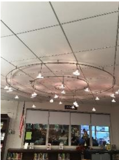
Image 11 Halogen Fixture
