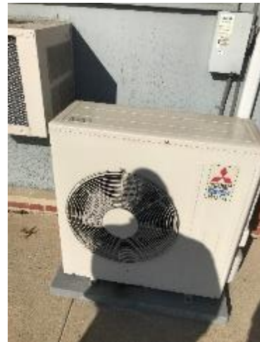
Image 20 Outdoor Condensing Unit
