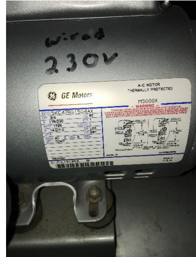
Image 15 Air compressor motor
