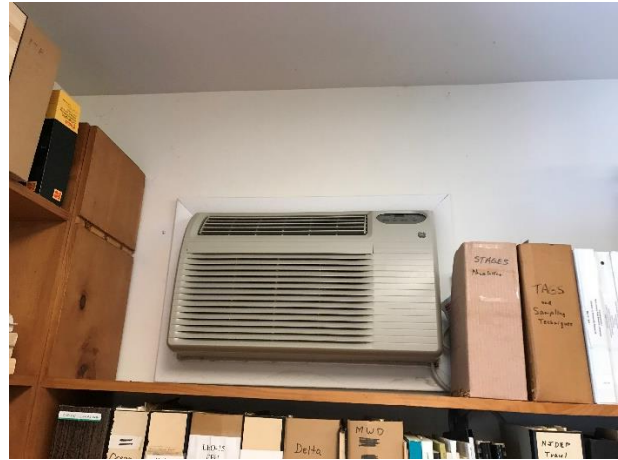
Image 9: Window AC in office
