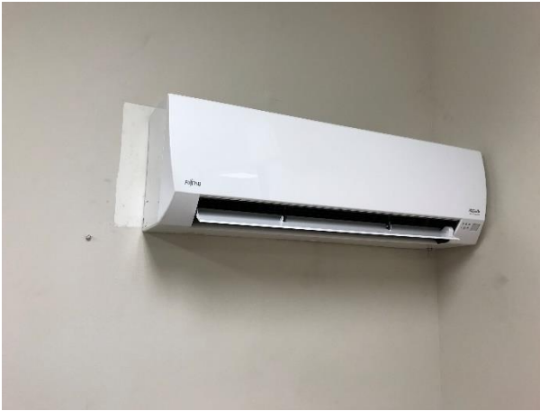
Image 8: Split system AC in vestibule
