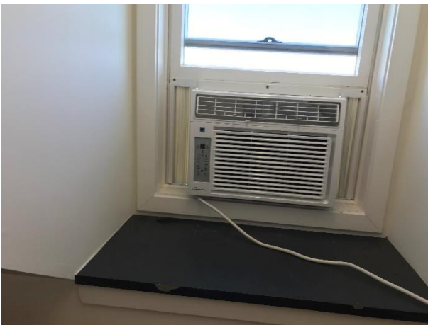
Image 6: Window AC in office
