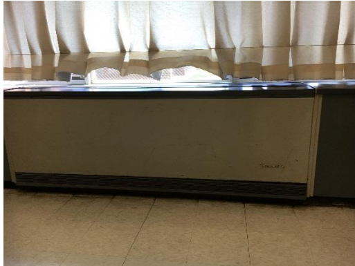
Original Unit Ventilator
