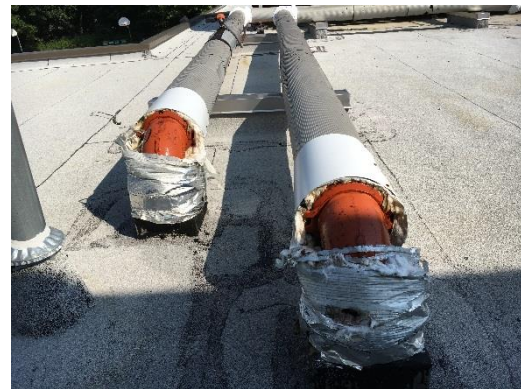
Chilled water piping in poor condition
