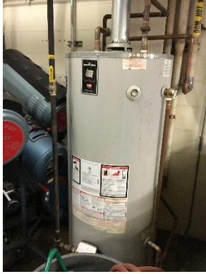
Storage Tank Water Heater
