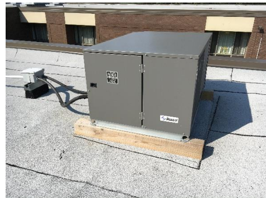
Walk-in equipment compressors
