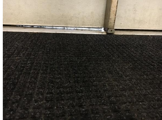
Exterior Door with worn weather-stripping
