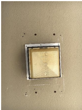
Surface mounted HID Canopy fixture
