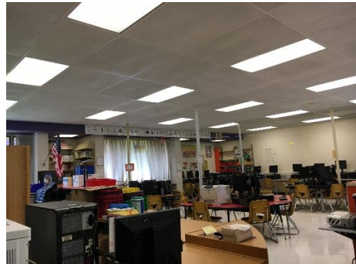
Recessed troffer fixtures
