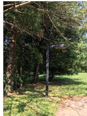
Pole mounted HID Shoebox fixture
