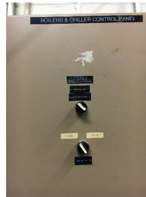
Boiler vs. chiller control switch
