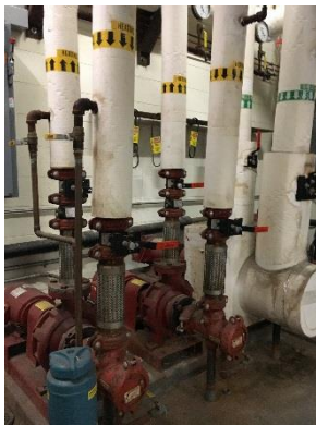
Hot water pumps and motors
