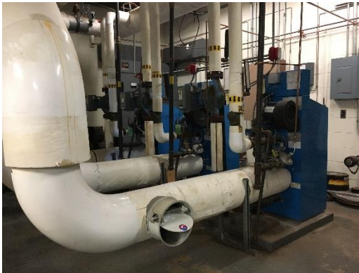
Condensing hot water boilers
