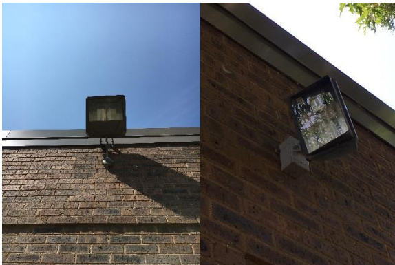
Wall mounted HID Flood fixtures
