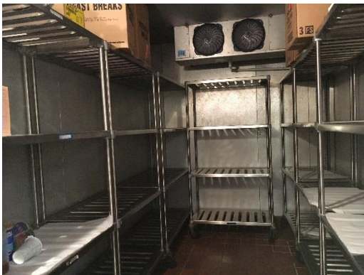
Walk-in cooler evaporator
