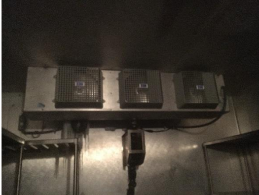
Walk-in freezer evaporator
