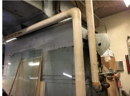
AHU with Hot/Chilled Water Coil
