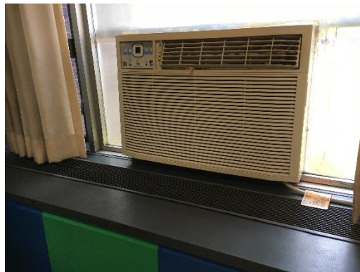
Window AC unit
