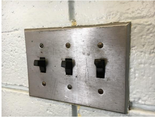
Typical Bi-Level Switching in Classrooms
