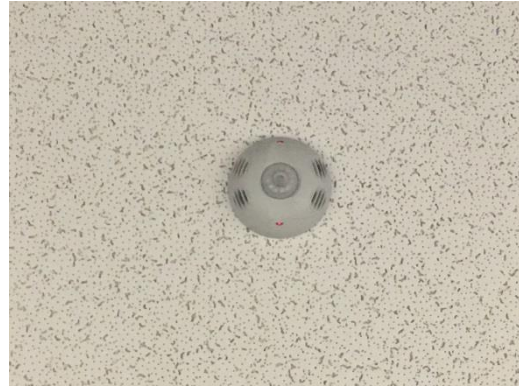
Typical Ceiling Mounted Occupancy Sensor
