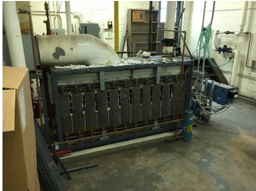
Non-Condensing Hot Water Boiler
