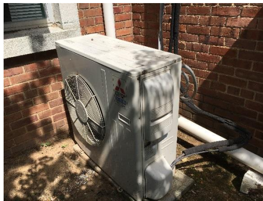
Split HP System – Outdoor Condensing Unit
