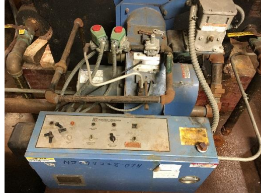
Boiler Burner
