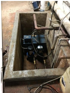
Condensate Return Pump Motors
