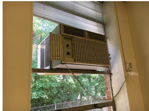
Window AC Unit
