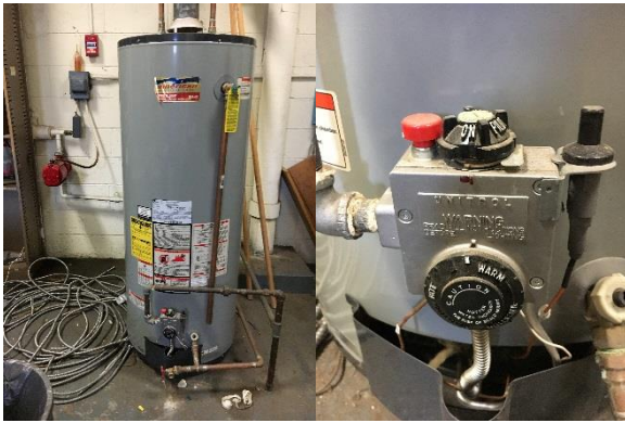
Storage Tank Water Heater & Tank Temperature Dial
