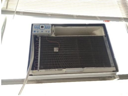
Window AC Unit in Poor Condition
