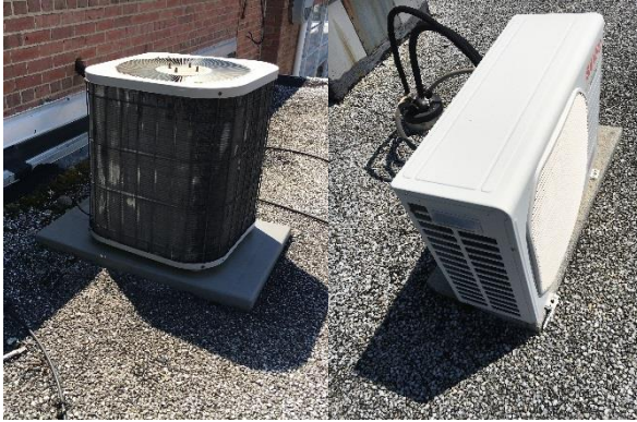
Split AC System – Outdoor Condensing Units
