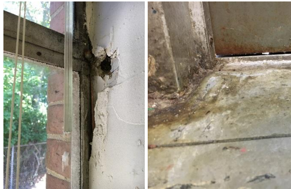
Building Envelope Deficiencies
