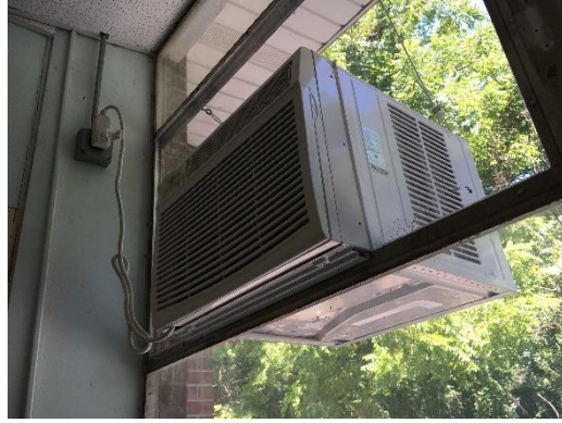
Window AC Unit
