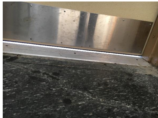
Exterior Door with no Weather-Stripping
