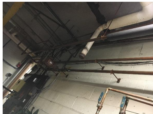
Basement Boiler Room - Uninsulated Piping
