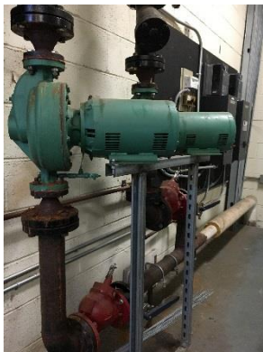
New Hot Water Pumps and Motors
