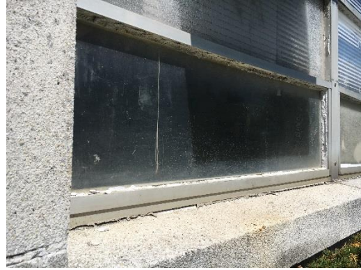
Window Frame Caulk in Poor Condition
