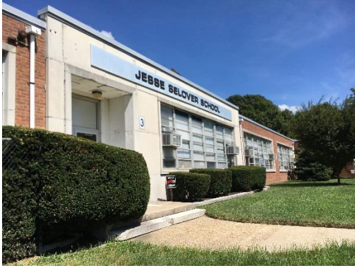
Building Façade – Old Entrance
