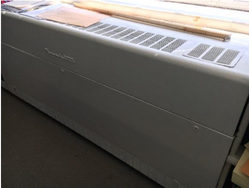
Old Unit Ventilator (UV)
