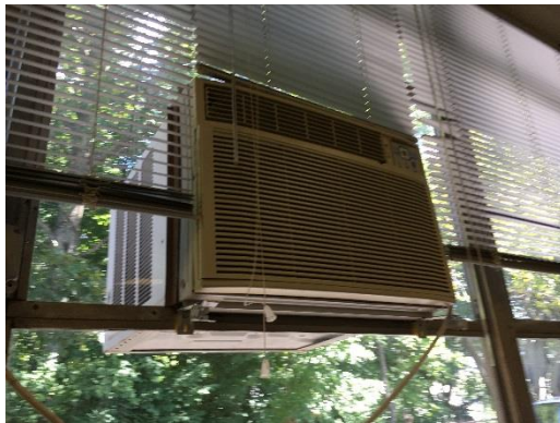
Window AC Unit
