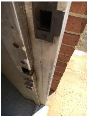
Exterior Door with no Weather-Stripping
