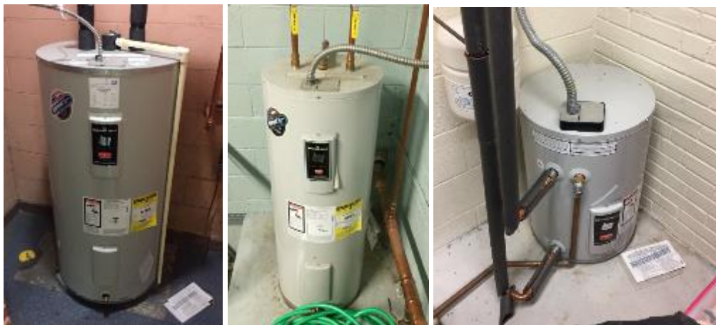
Image 8: DHW water heaters
