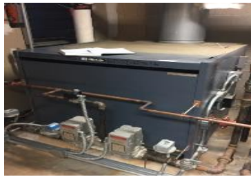
Image 5: Typical Hot Water Boiler
