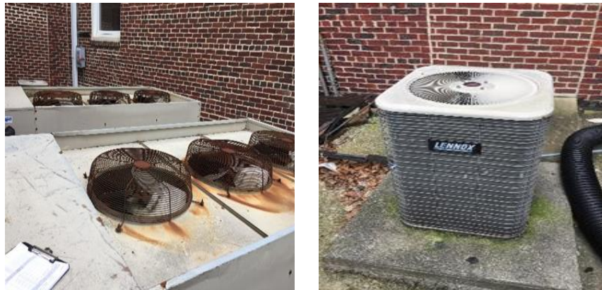
Image 5: Direct Expansion Air Conditioning System
