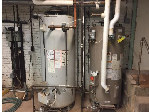
Image 6: Domestic Hot Water Heating System
