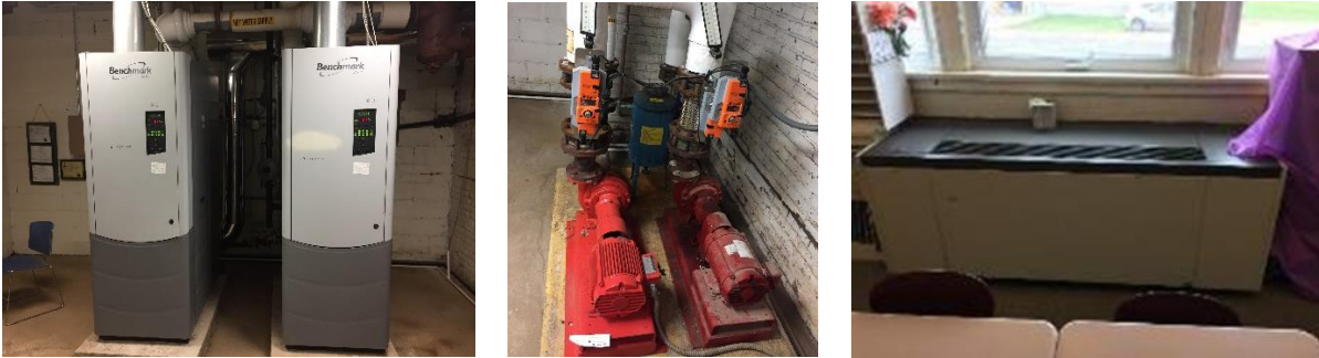
Image 4: Hot water heating system
