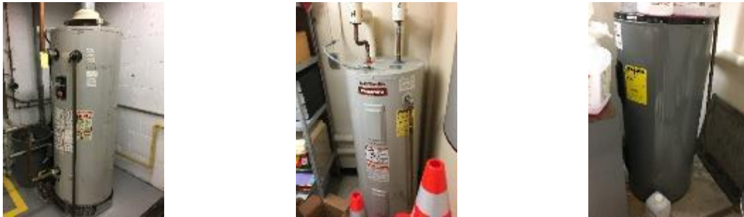
Figure 13 – Domestic Hot Water Equipment
