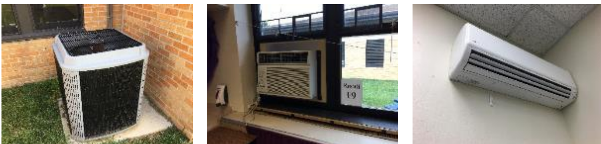
Figure 12 – Air Conditioning Equipment
