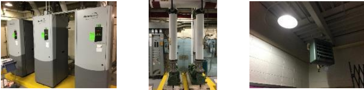
Figure 9 – Heating Hot Water Equipment
