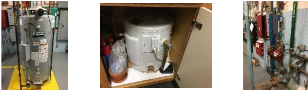
Figure 12 – Domestic Hot Water Equipment
