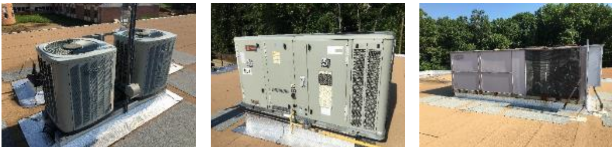
Figure 10 – Air Conditioning Equipment
