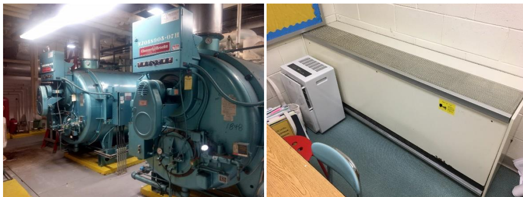
Image 3 Hot Water Heating System
