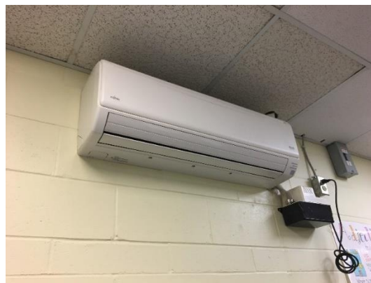
Image 5 Direct Expansion AC System
