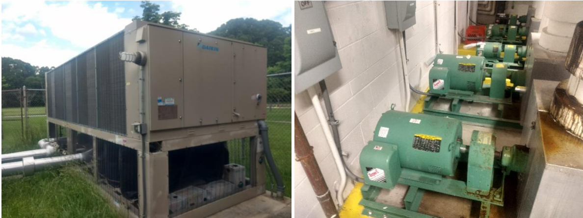
Image 4 Chilled Water Air Conditioning System
