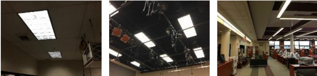
Figure 8 – Interior Lighting Technologies
