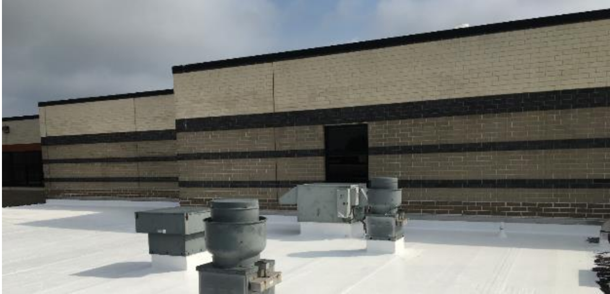
Figure 7 – Roof with New Reflective Surface
