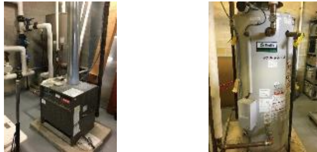
Figure 11 – Domestic Hot Water Equipment
