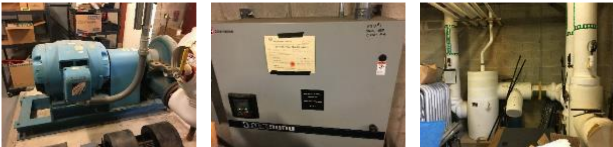
Figure 9 – Heat Pump Water Loop Equipment
