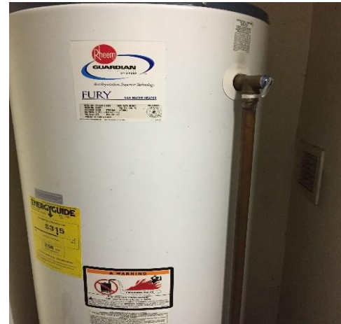
Domestic hot water unit
