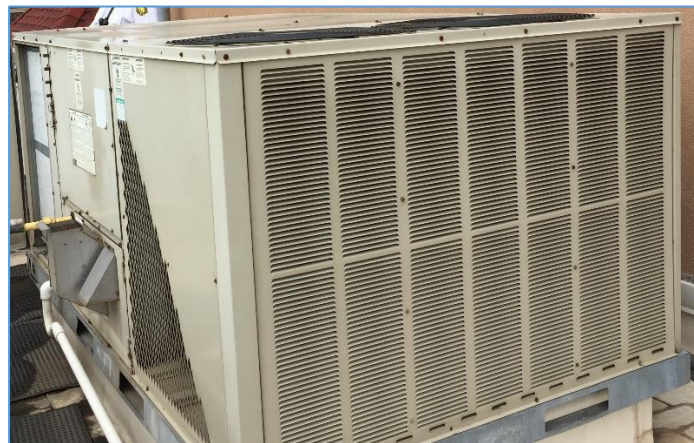
Rooftop air handling unit
