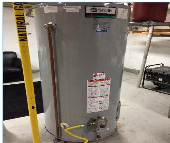
Domestic hot water heater
