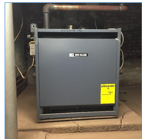
Weil McLain boiler at the basement
