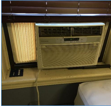
Window AC in the dormitory
