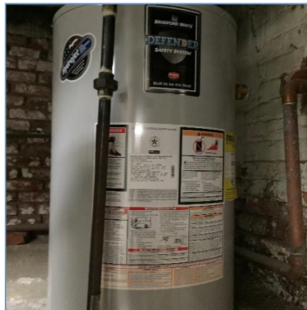
Bradford White domestic hot water heater unit
