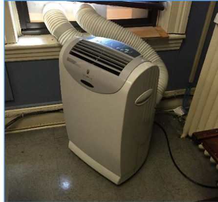
Plug in air-cooler in the dormitory
