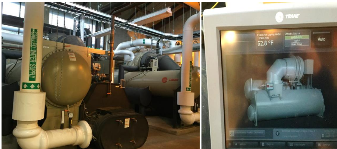
Image 2: Central Chiller System
