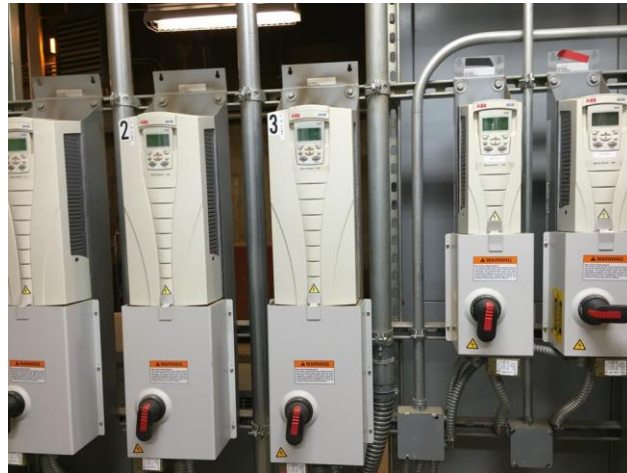
Image 4: All large motors in the Central Utility Plant are controlled by VFDs
