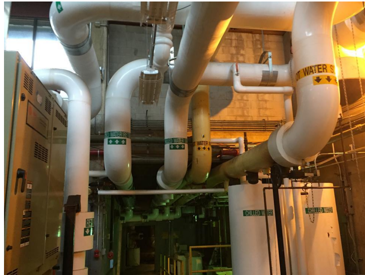
Image 1: Campus-Wide Hot and Chilled Water Distribution Systems
