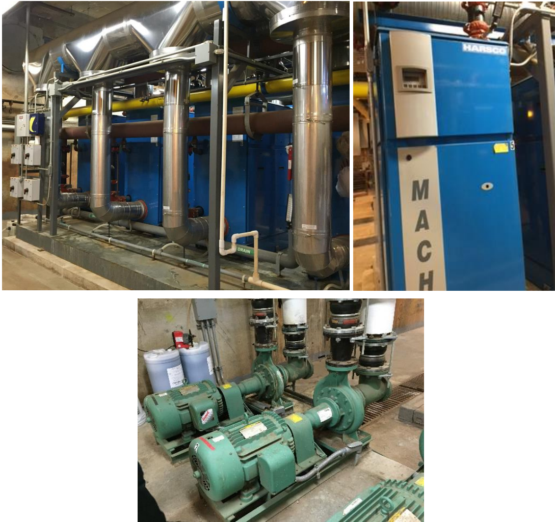
Image 3: Campus main boiler system & heating hot water pump
