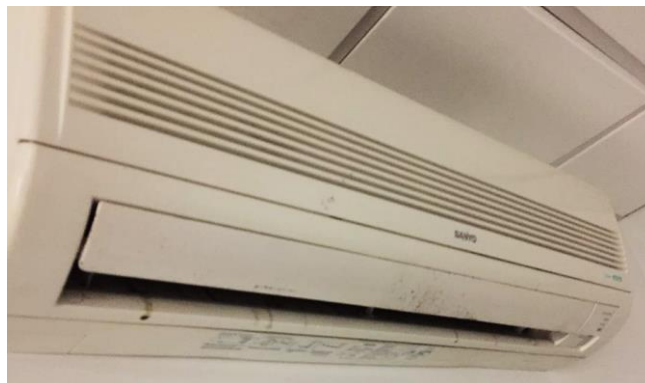
Image 5: Ductless mini-split heat pump in office area
