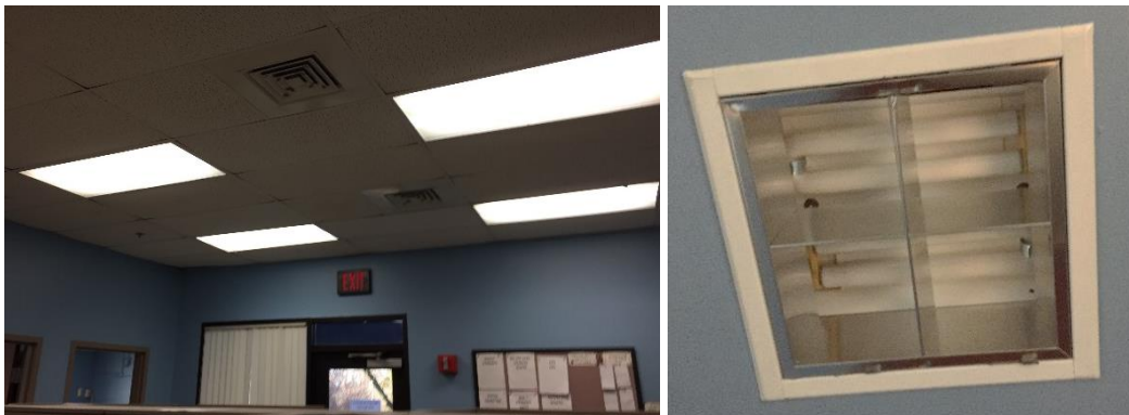
Image 2: Building Interior & Exterior Lighting
