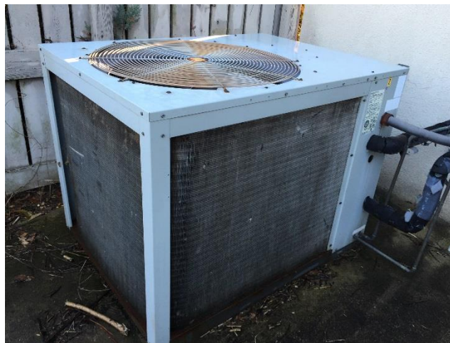
Image 3: Split System Condenser and HVAC Controls
