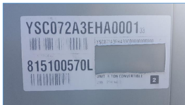
Nameplate of the HVAC rooftop unit
