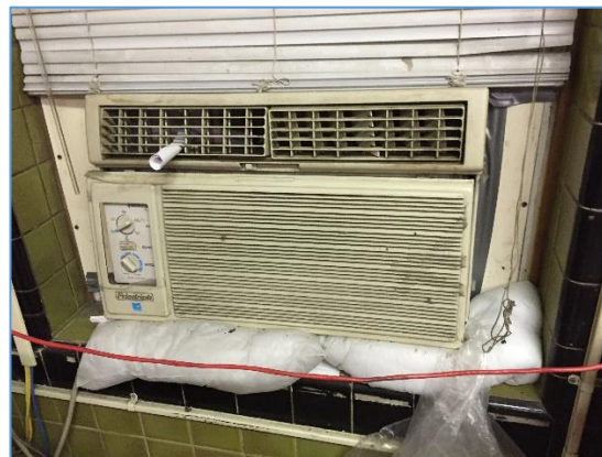
Right: Non-functional AC unit in the reception area
