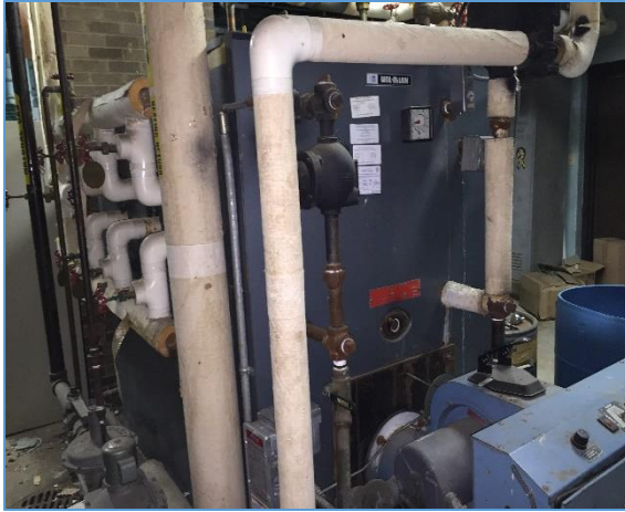
Weil-McLain Boiler (Left); Warm Air Unit heater (Right)
