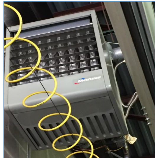
Warm air unit heater in the apparatus floor
