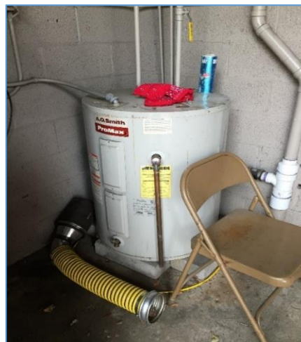
Electric domestic water heater
