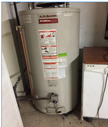
Natural Gas fired water heater (74 gallon)
