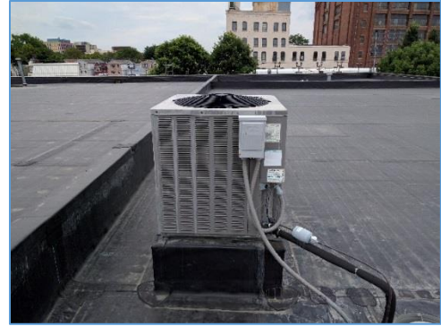
Condensing unit on the rooftop
