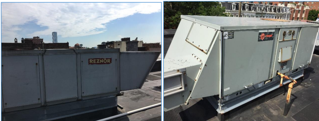
Reznor air handling unit (left); Trane air handling unit - rooftop of the firehouse (right)
