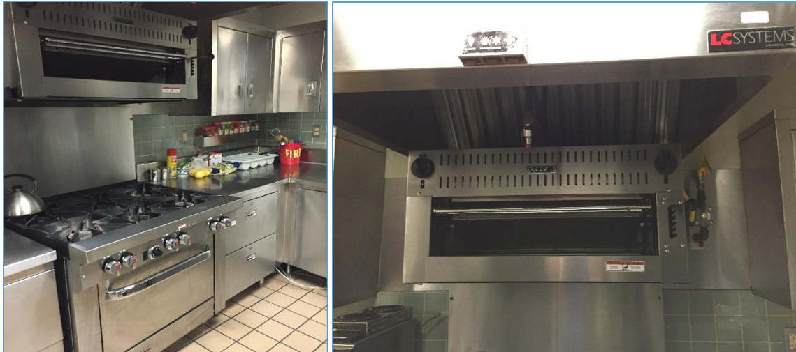
Kitchen Equipment – Burners, Oven and Griddle
