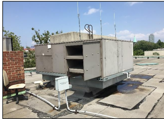
Roof top air handling unit
