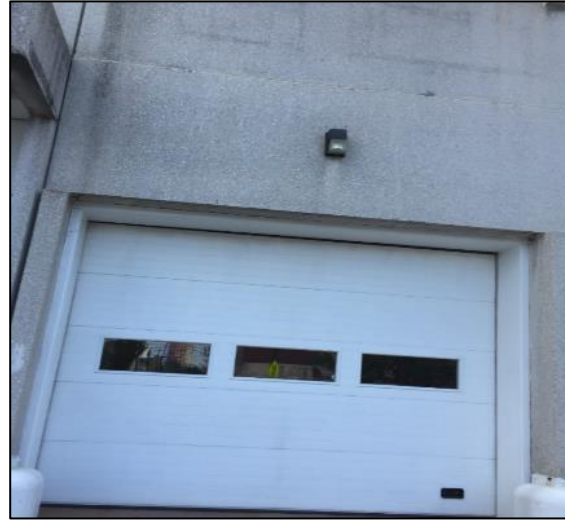
Figure 7 - Exterior Walls and Garage Door
