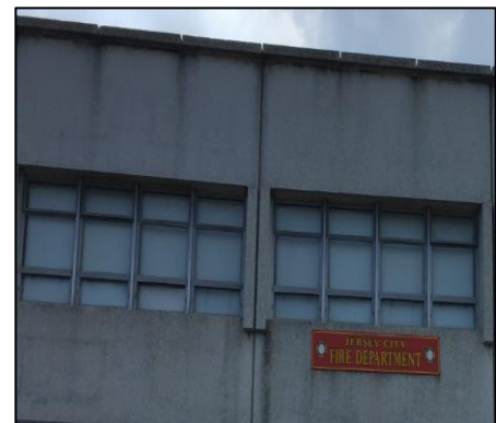
Figure 6 - Exterior Walls and Windows
