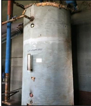
Domestic hot water heater
