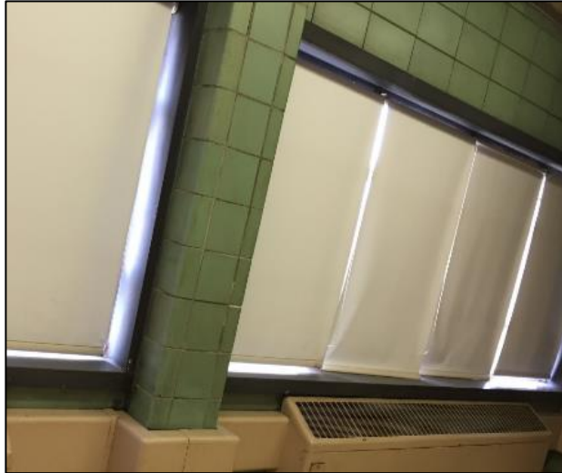
Figure 8 - Interior walls and windows
