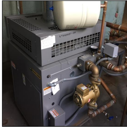
Weil Mclain boiler
