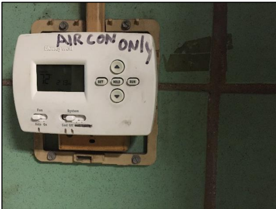
Thermostat in the first floor
