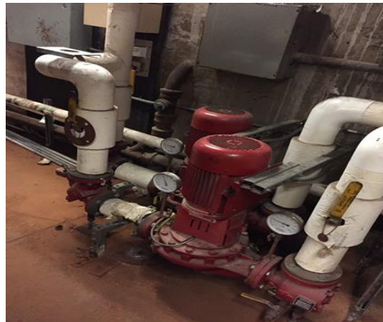
Image 2: Steam to Hot Water Heating System
