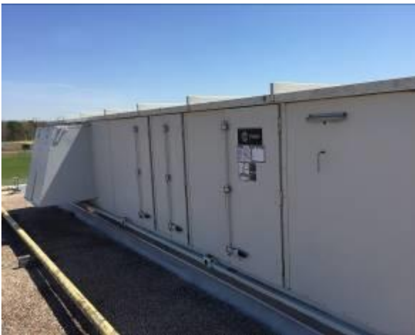
Image 9 – AHU-1 (New Wing)
