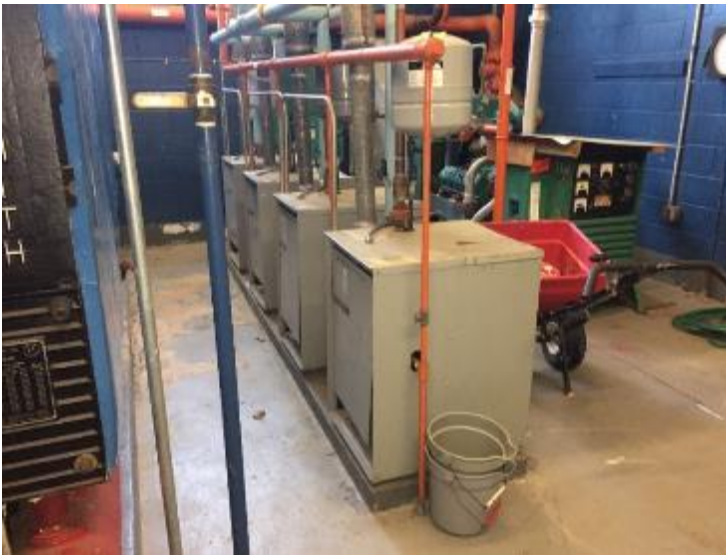
Image 15 - Modular Boilers (DHW)
