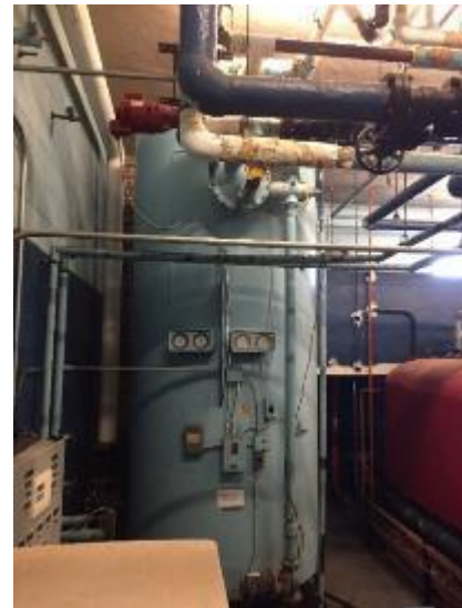
Image 16 – DHW Storage Tank
