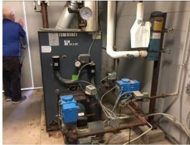
Image 8 – New Wing Boiler
