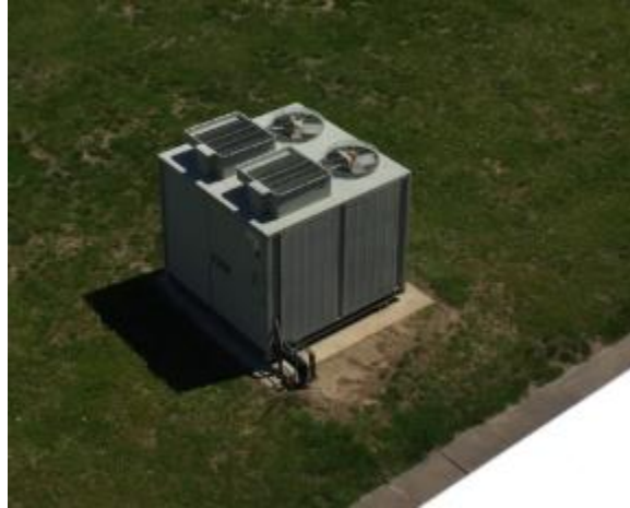
Image 5 – New Wing Chiller
