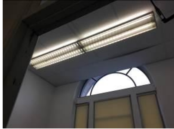
Image 4 – Saybrook Annex T8 Fluorescent Lighting
