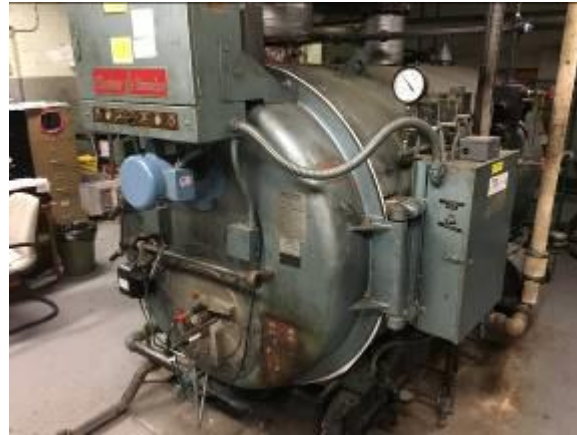
Image 6 – Saybrook Annex Steam Boiler
