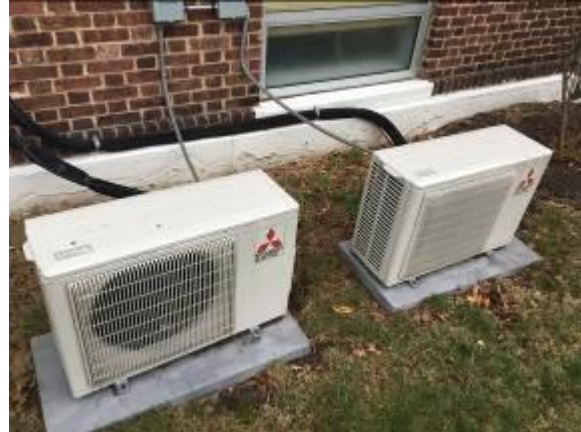
Image 8 – Saybrook Annex Split HP Outdoor Coil Units
