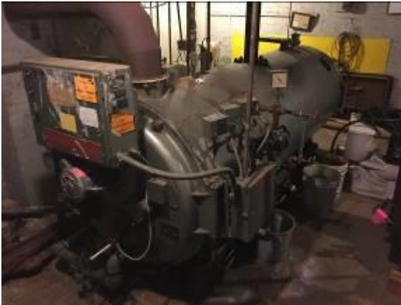
Image 5 – Admin. Bldg Steam Boiler
