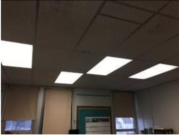
Image 3 – Admin. Bldg. T8 Fluorescent Lighting
