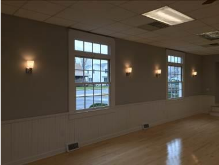
Image 3 – T8 Fluorescent Lighting (classroom-new section)
