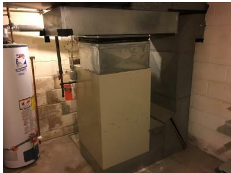
Image 6 – Split-System AC (supply fan/evaporator)
