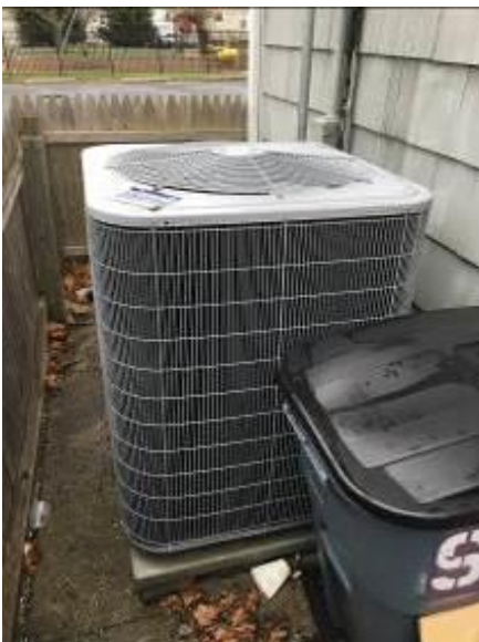
Image 5 – Split-System AC (condenser)
