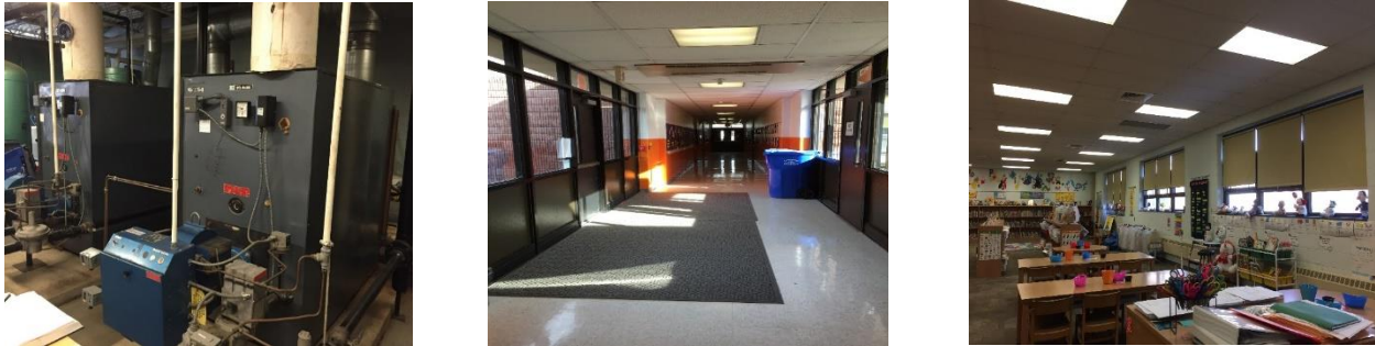
Image 3 Facility Boiler and terminal units
