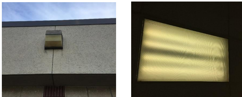
Image 2 Typical Lighting Fixtures
