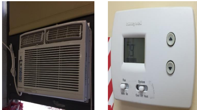
Image 4 Sample of AC systems and control units
