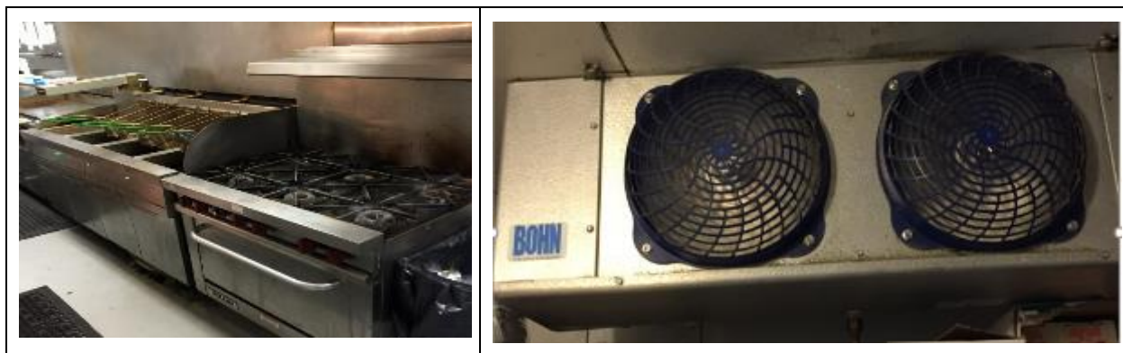
Image 14: Cafeteria Cooking equipment & Walk in Units
