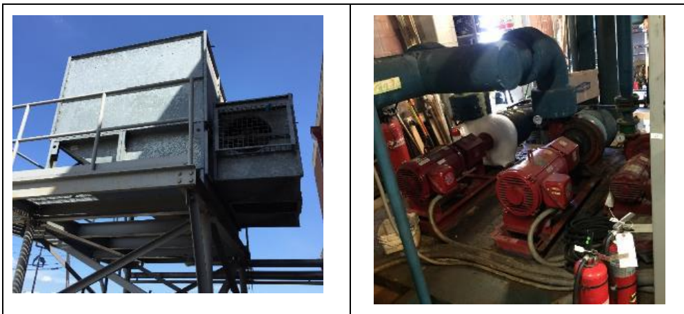
Image 7: Cooling Tower and Chilled Water Pumps
