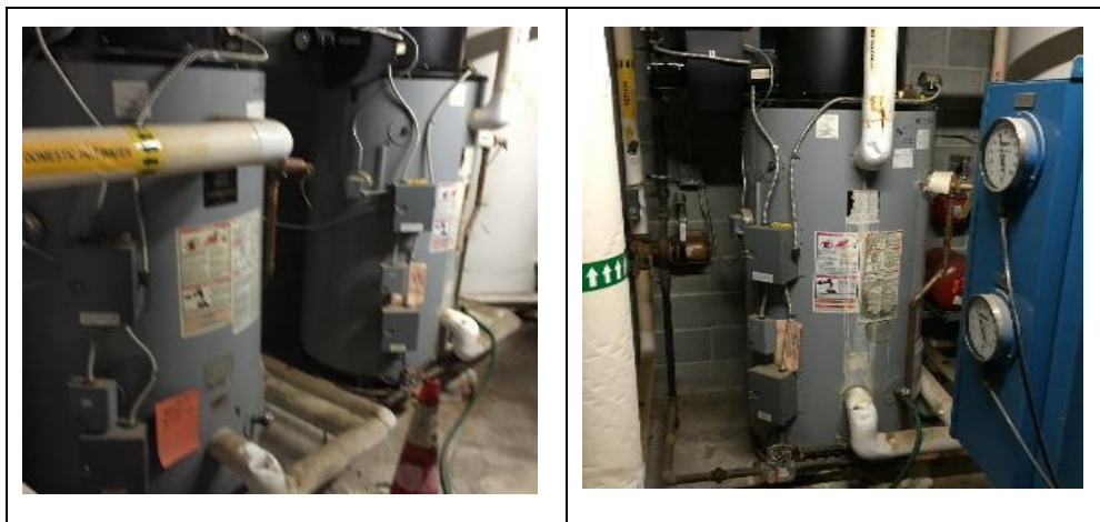
Image 13: Domestic Hot Water Systems
