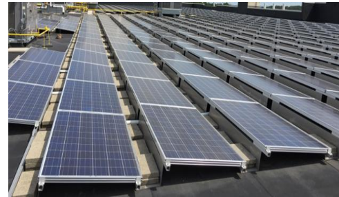
Image 3: Roof Mounted PV Arrays
