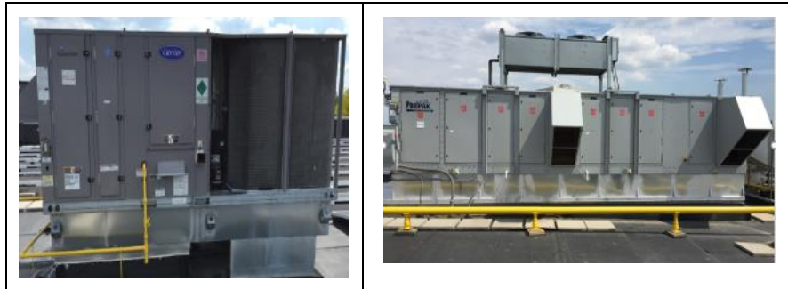
Image 9: Roof Top Units
