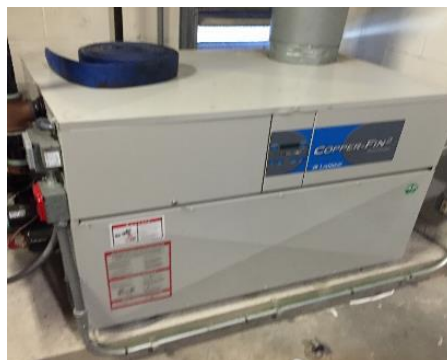
Image 8: Pool Hot Water Boiler
