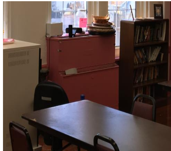
Image 6 Radiator in Classroom
