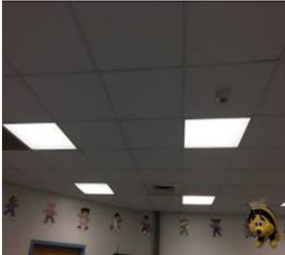
Image 3 – T8 Fluorescent Lighting (classroom-new section)
