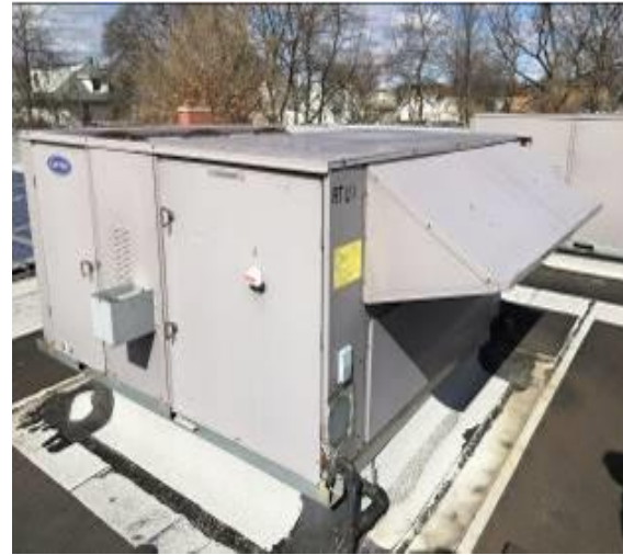
Image 8 – Package Terminal Unit (RTU1- serves classrooms)
