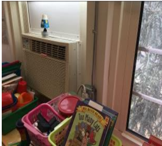
Image 7 – Window AC (Classroom 1)
