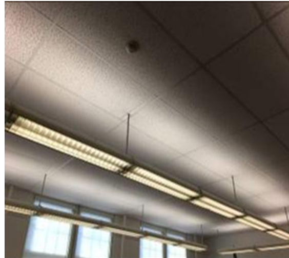
Image 4 – T8 Fluorescent Lighting (classroom-old section)
